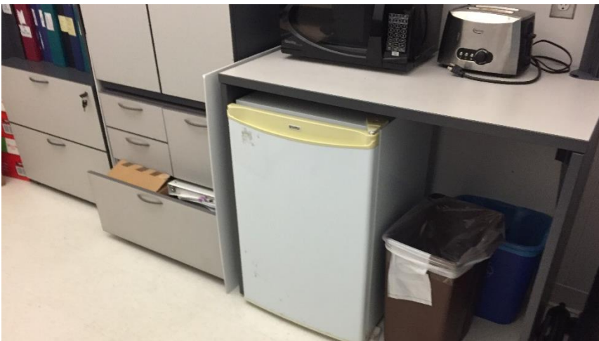
Photo 8: Representative view of the equipment containing ODSs observed throughout the subject building.
