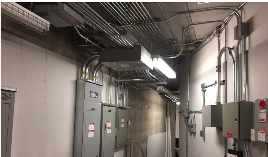
Photo 11: Representative view of the fluorescent light fixtures containing mercury vapour observed throughout the subject building.
