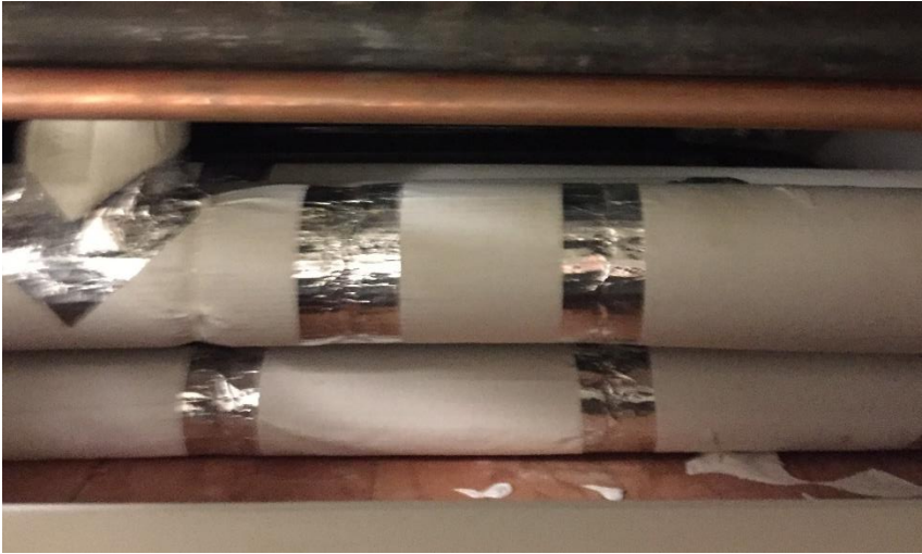
Photo 1: Representative view of the non-asbestos-containing mechanical insulation observed throughout the subject building.
