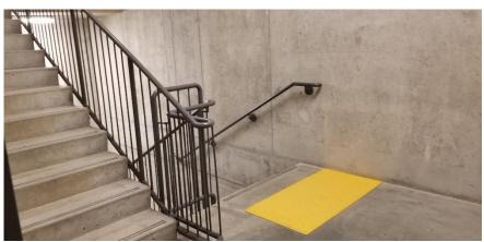
**Photo 10:** Typical silica containing concrete finishes.
