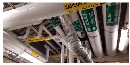
Photo 11: Typical view of fibreglass mechanical insulation throughout the subject building.
