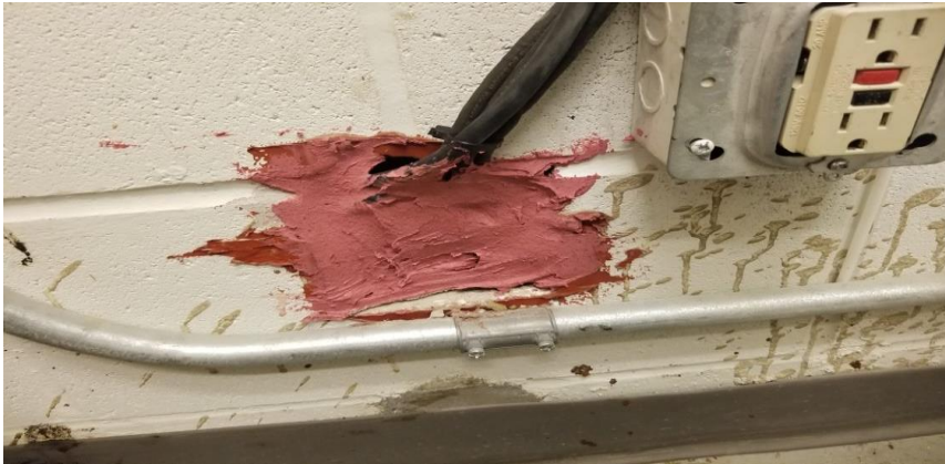
Photo 13: View of non-asbestos containing firestop caulking (Pink) observed in Room 0027F.
