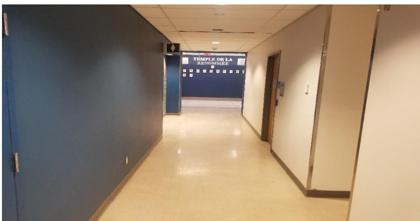
Photo 3: View of typical hallway finishes with lead-acid batteries present in emergency lights.
