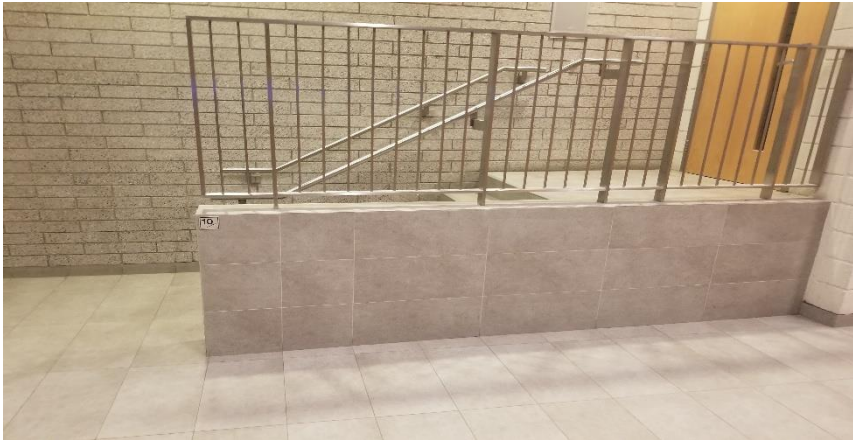
Photo 4: Typical silica contains brick, mortar, concrete, and ceramic tile finishes.
