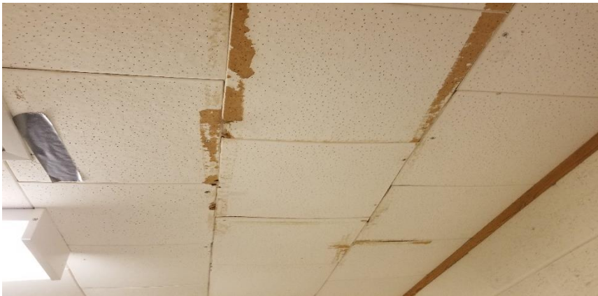
Photo 14: View of non-asbestos screwed on ceiling tiles observed in Room E018B.
