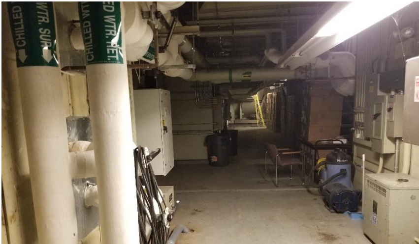
Photo 1: Representative view of the finishes observed throughout Room 600.
