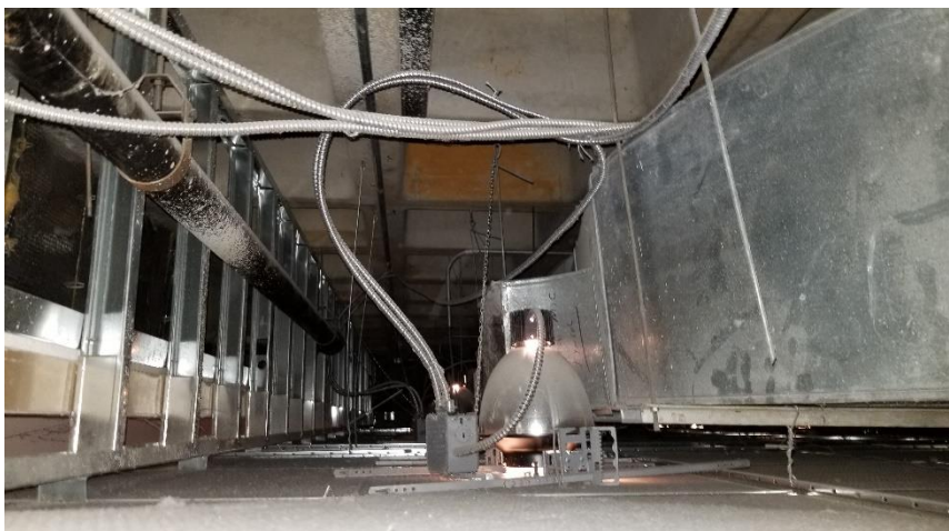
Photo 26: Representative view of the ceiling space in Room 147B.
