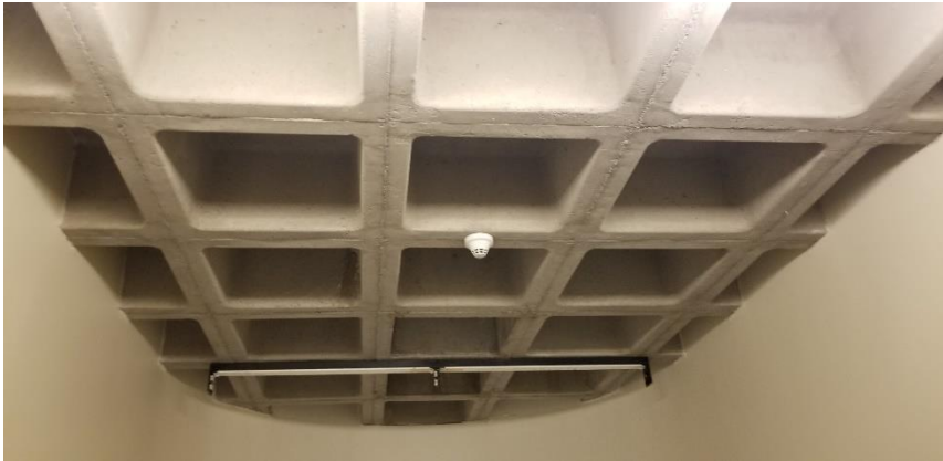
Photo 13: View of the concrete ceilings observed throughout the subject building.
