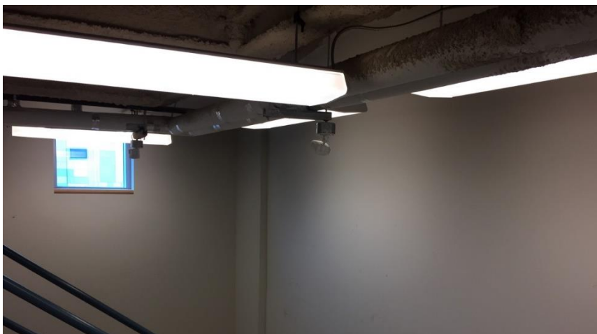
Photo 8: Representative view of the mercury-containing fluorescent light fixtures observed throughout the subject building.
