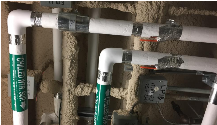
Photo 5: View of the non-asbestos sprayed fireproofing observed throughout the subject building.
