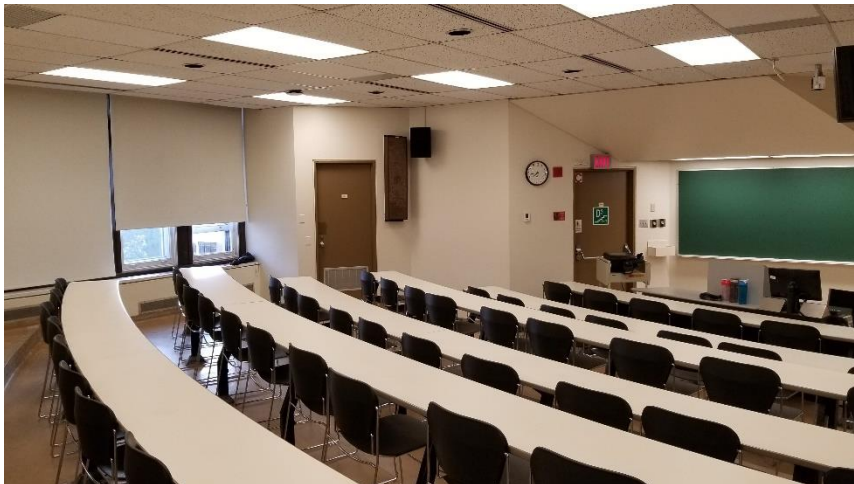
Photo 13: Representative view of the classroom finishes observed throughout the 3 rd Floor.
