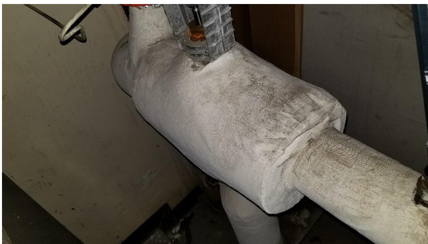
Photo 12: View of the fiberglass mechanical pipe fitting and pipe straight insulation observed throughout the subject building.
