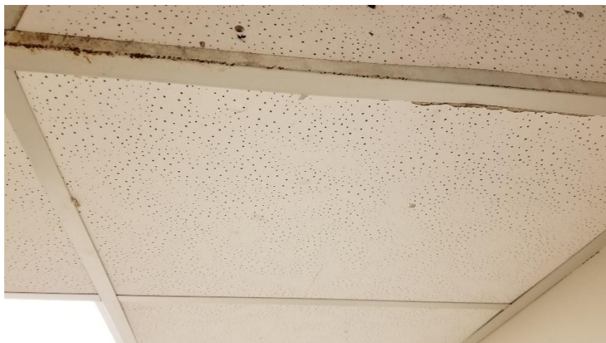
Photo 16: View of the asbestos-containing ceiling tiles (2'x4' White w/ Small Pinholes) observed in Room 106.
