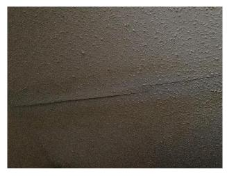
Photo 4: View of water damaged ceiling texture coat observed in apartment 198 - bedroom of 620 King Edward
