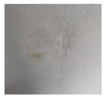
Photo 5: View of water damaged ceiling texture coat observed in apartment 196 – living room of 620 King Edward
