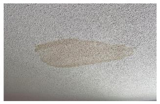
Photo 7: View of water damaged ceiling texture coat observed in apartment 187 – living rooms of 75 Louis-Pasteur
