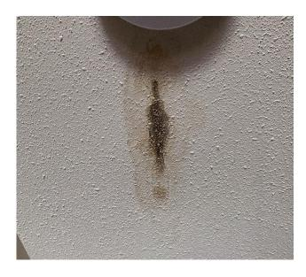
Photo 8: View of water damaged ceiling texture coat observed in apartment 184 - hallway of 75 Louis-Pasteur
