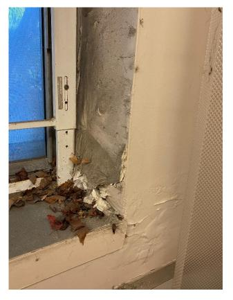
Photo 8: View of water damaged window sill observed in the basement laundry room of 624 King Edward
