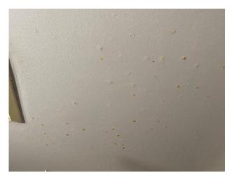
Photo 11: View of mould observed in apartment 155 – full bath ceiling of 622 King Edward
