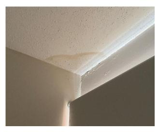
Photo 12: View of water damaged ceiling texture coat observed in apartment 151 - bedroom of 622 King Edward
