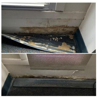
Photo 2: View of water damaged drywall wall observed in apartment 180 - living room of 79 Louis-Pasteur
