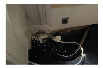
Photo 13: View of water damaged drywall wall observed in apartment 152 – living oom of 622 King Edward
