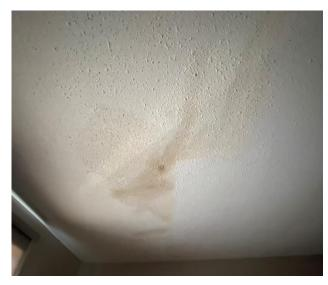
Photo 4: View of water damaged ceiling texture coating observed in apartment 173 – dining room of 79 Louis-Pasteur
