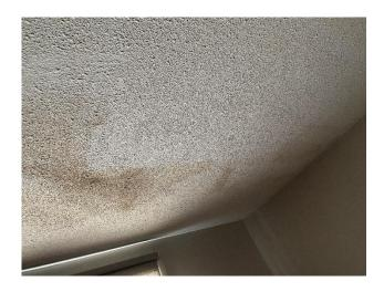
Photo 3: View of water damaged ceiling texture coating observed in apartment 177 – living room of 79 Louis-Pasteur
