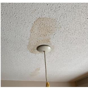
Photo 9: View of water damaged ceiling texture coat observed in apartment 157 – dining room of 624 King Edward
