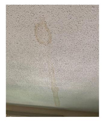
Photo 6: View of water damaged drywall wall observed in apartment 168 living room of 624 King Edward
