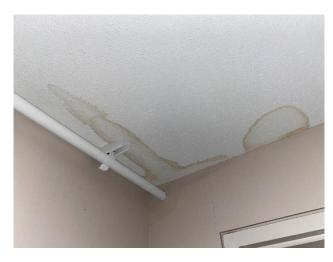
Photo 3: View of water damaged ceiling texture coat observed in apartment 73 doorway of 630 King Edward
