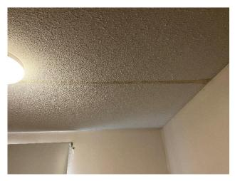
Photo 2: View of water damaged ceiling texture coat observed in apartment 76 – bedroom of 630 King Edward
