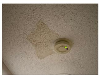
Photo 5: View of water damaged ceiling texture coat observed in apartment 90 – hallway of 632 King
