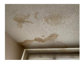
Photo 1: View of water damaged ceiling texture coat observed in apartment 81 – living room of 630 King Edward
