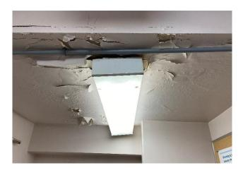
Photo 3: View of water damaged ceiling drywall observed in the basement laundry room of 101 Louis-Pasteur
