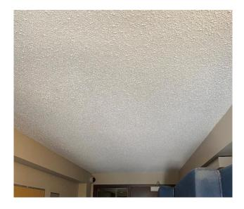
Photo 1: View of non-asbestos containing ceiling texture coat observed throughout the buildings
