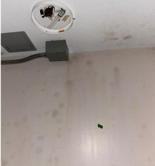
Photo 4: View of mould observed in apartment 51 – hot water tank storage closet of 634 King
