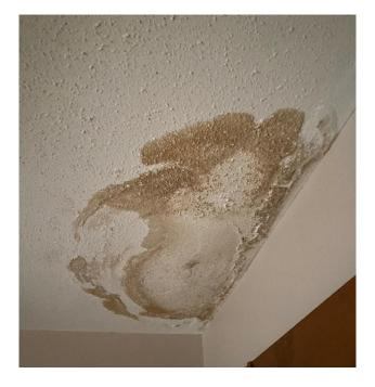
Photo 11: View of water damaged ceiling texture coat observed in apartment 35 – bedroom of 85 Marie Curie
