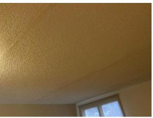
Photo 10: View of water damaged ceiling texture coat observed in apartment 19 – living room of 95 Marie Curie
