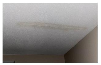
Photo 3: View of water damaged ceiling texture coat observed in apartment 9 - dining room of 638 King Edward
