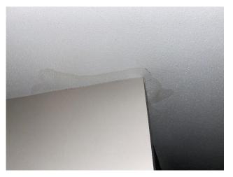
Photo 6: View of water damaged ceiling texture coat observed in apartment 1 bedroom of 638 King Edward
