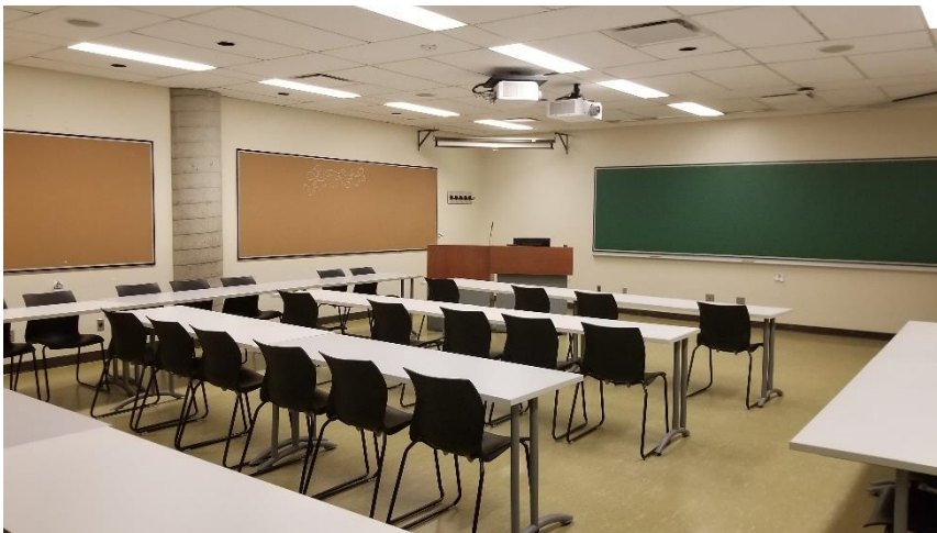
Photo 27: Representative view of the finishes observed throughout Room 407, including asbestos-containing vinyl floor tiles (12"x12" Green w/ White Striped) observed in good condition.
