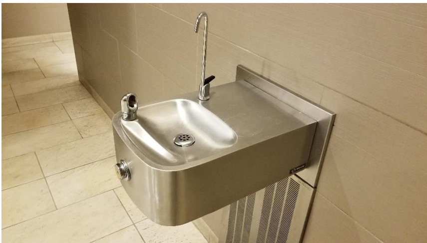
Photo 12: View of the equipment containing ODSs observed in Room C100A.
