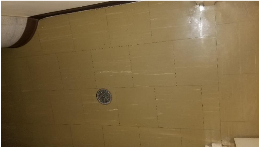
Photo 28: View of the asbestos-containing vinyl floor tiles (12"x12" Green w/ White Striped) observed in good condition in Room 471.
