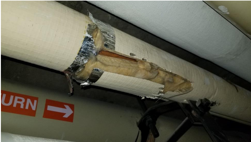
Photo 5: View of the non-asbestos containing pipe straight insulation observed throughout Room 01.
