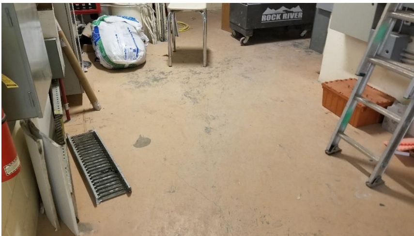
Photo 15: View of the floor paint (Pink) in Room 104A, which was determined not to contain lead.
