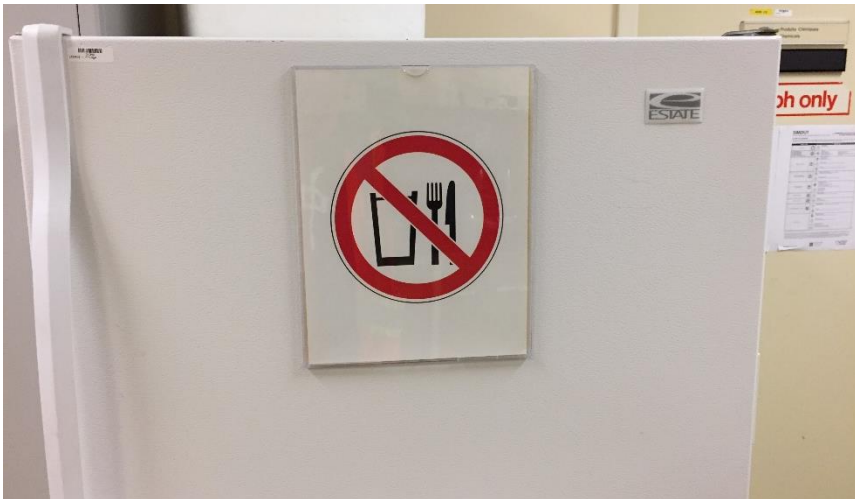
Photo 29: View of the equipment containing ODSs observed in Room 402.
