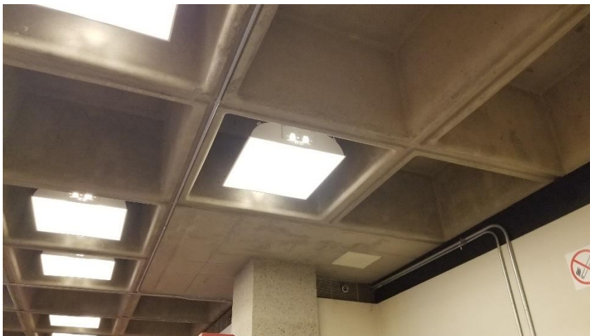
Photo 2: Representative view of the concrete ceilings observed throughout the 0 Level.
