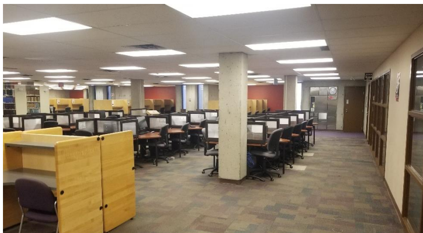
Photo 32: Representative view of the finishes observed throughout Level 6.
