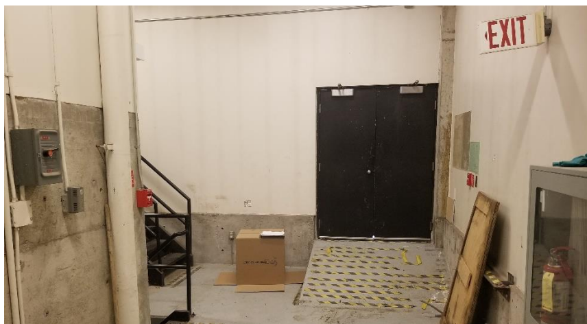
Photo 33: Representative view of the finishes observed in Room 703A.
