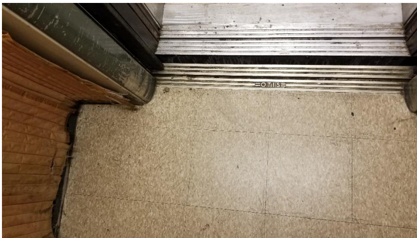
Photo 5: View of the non-asbestos vinyl floor tiles (12"x12" - Brown w/ White Spots) were observed and sampled in Room 007D.
