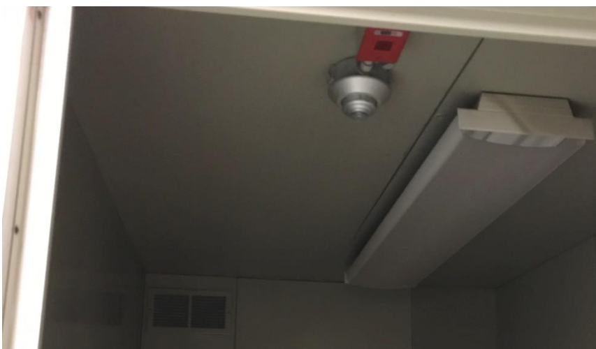
Photo 3: Typical view of the fluorescent light fixtures containing mercury vapour.
