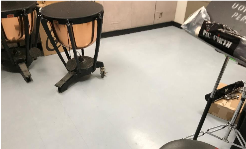
Photo 1: Representative view of the previously identified asbestos-containing VFT 12"x12" Green/Blue in Room 106, 109A, containing 1% Chrysotile asbestos.
