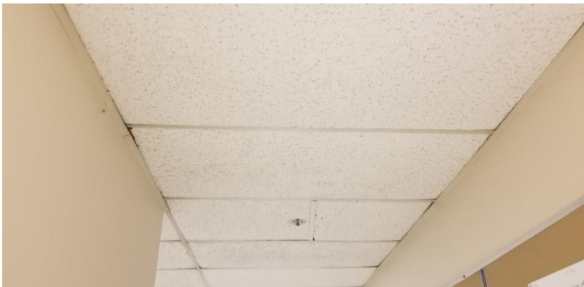
Photo 6: View of the non asbestos-containing ceiling tiles observed throughout Level 00.
