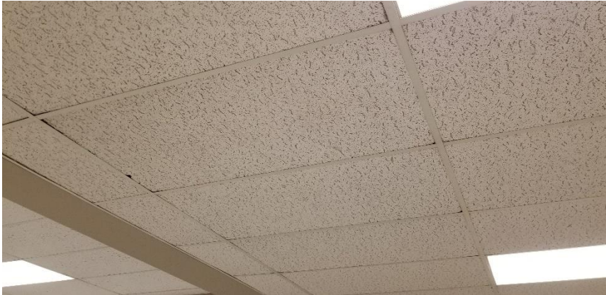
Photo 7: View of the non asbestos-containing ceiling tiles observed throughout Level 00.
