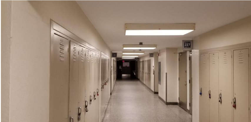
Photo 19: Representative view of the hallway finishes observed throughout Level 2.
