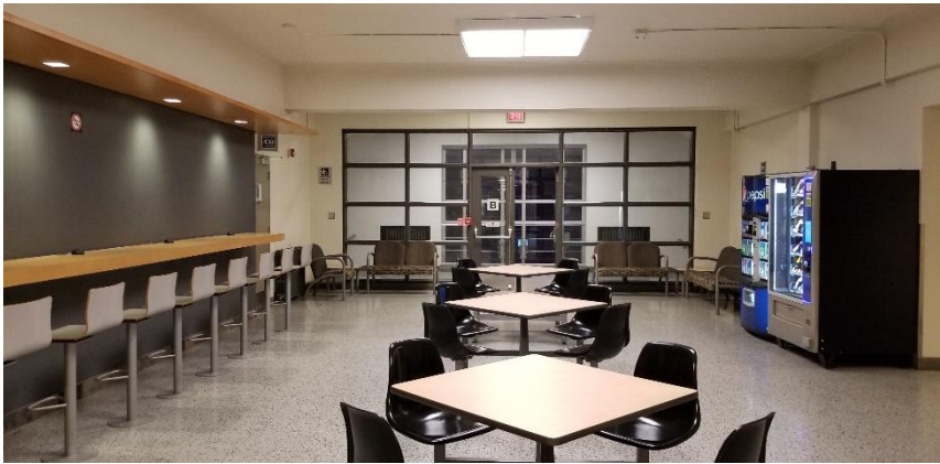
Photo 2: Representative view of the common area finishes observed throughout the subject building.
