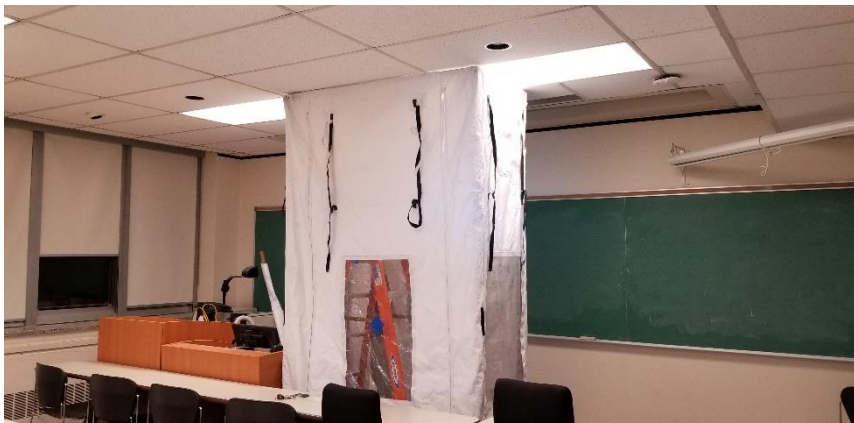
Photo 29: Representative view of the Type 2 ceiling entries performed during the site survey to access ceiling spaces.
