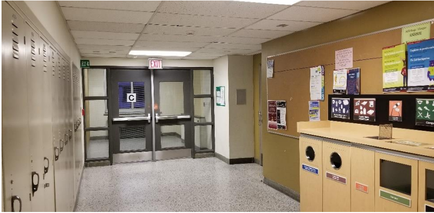
Photo 1: Representative view of the hallway finishes observed throughout the subject building.
