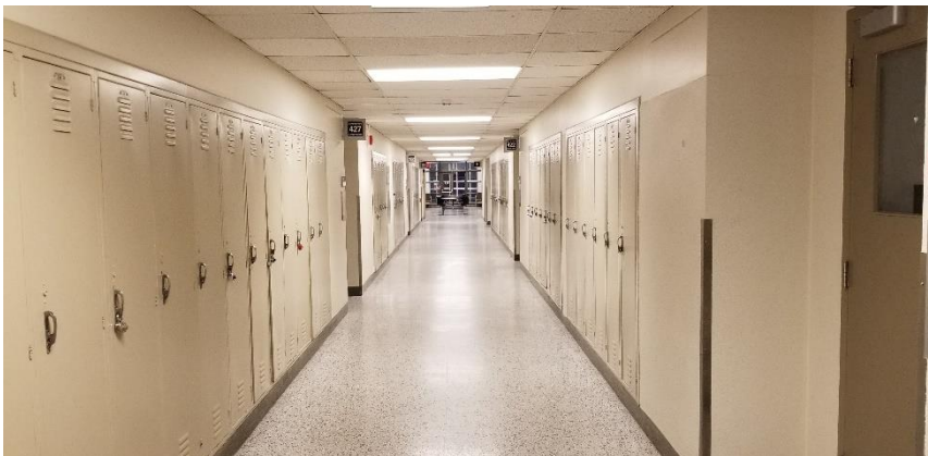
Photo 3: Representative view of the hallway finishes observed throughout the subject building.
