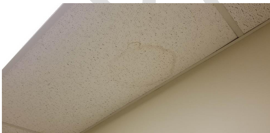
Photo 6: View of water stained asbestos-containing ceiling tiles (2'x4"-White Tone) observed in Room W0011B.
