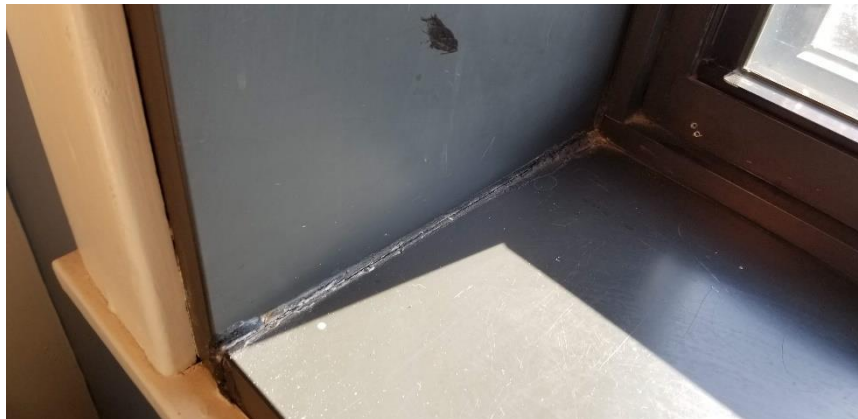
Photo 13: View of asbestos-containing window frame caulking observed to be in fair condition in Room M386F.
