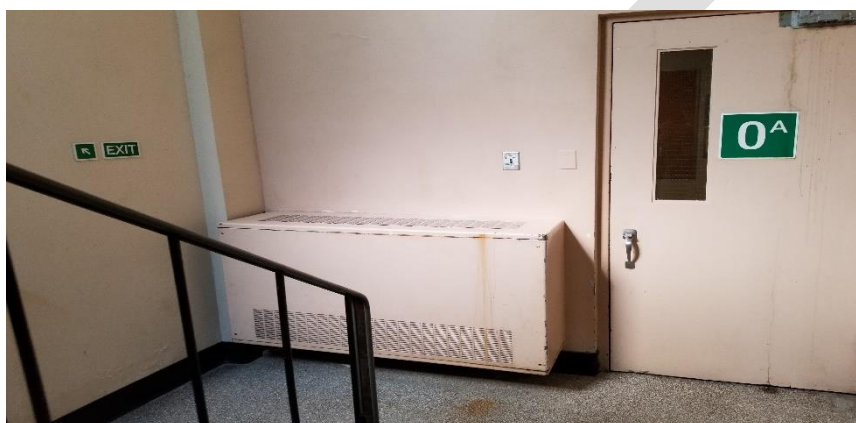
Photo 20: Typical view of low-level lead containing pink paint finish observed to be in good condition on radiators and walls throughout the subject building.
