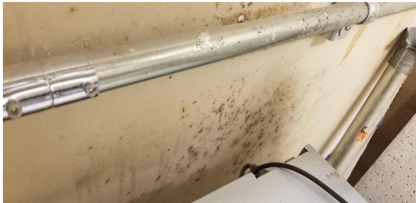
Photo 16: View of mold impacted drywall observed in Room N0109.
