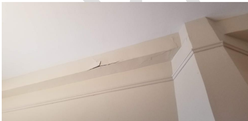
Photo 12: View of asbestos-containing ceiling plaster observed to be in poor condition in Room M386.
