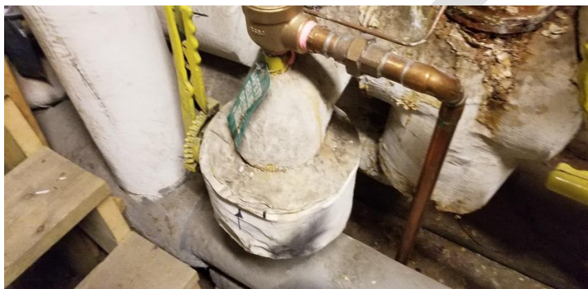
Photo 8: View of asbestos-containing mechanical pipe fitting insulation observed to be in good condition in Room C01B.
