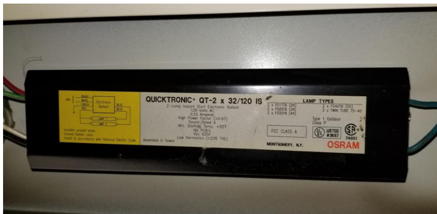
Photo 19: View of non-PCB Containing light ballasts observed in C459.
