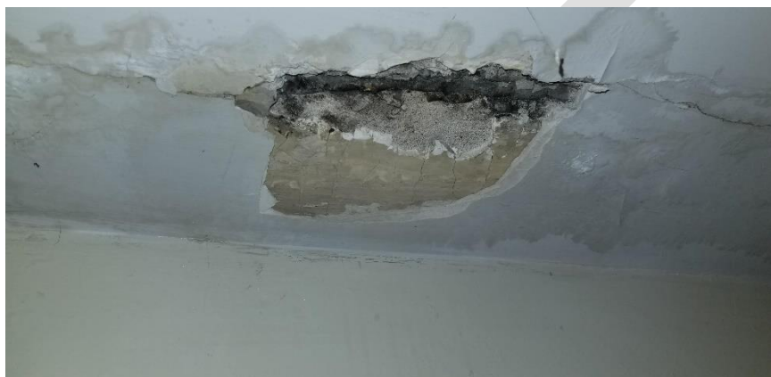
Photo 11: View of asbestos-containing ceiling plaster observed to be in poor condition in Room C401A.
