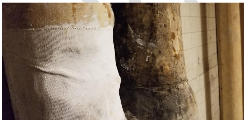
Photo 15: View of mould and water damage observed on pipe fittings and straights in Room C01D.
