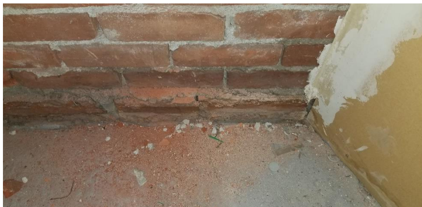
Photo 7: View of the asbestos-containing brick mortar observed to be in poor condition in Room C455.
