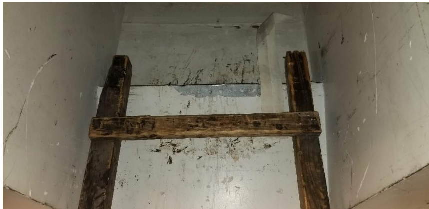
Photo 4: View of asbestos-containing drywall joint compound observed to be in poor condition in Room C452
