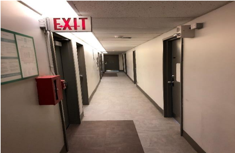
Photo 1: View of typical finishes observed at the building located at 45 University Private.
