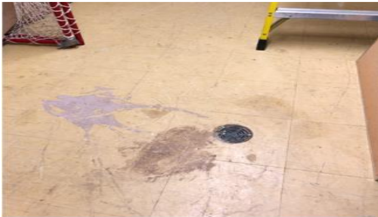
Photo 5: View of asbestos-containing vinyl floor tiles (12"x12" - Yellow) observed in Room 012.
