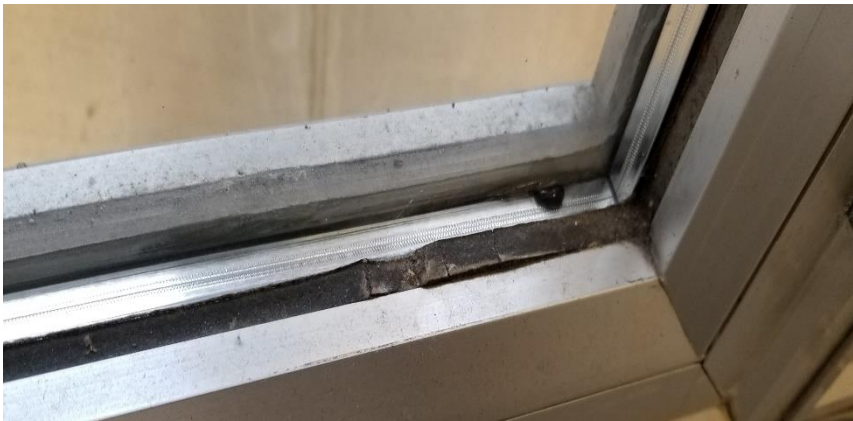
Photo 2: View of asbestos-containing window caulking observed to be in good condition in Room 1070 and other stairwells throughout the subject building.
