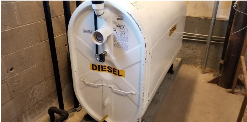
Photo 10: View above ground storage tank observed to be in good condition in Room 7028A.
