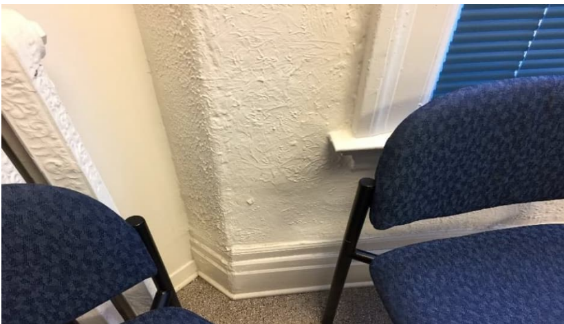
Photo 5: View of the non-asbestos-containing texture coat observed on the walls in Room 18.
