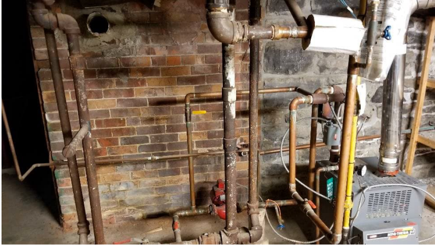
Photo 1: Typical view of finishes in the basement.
