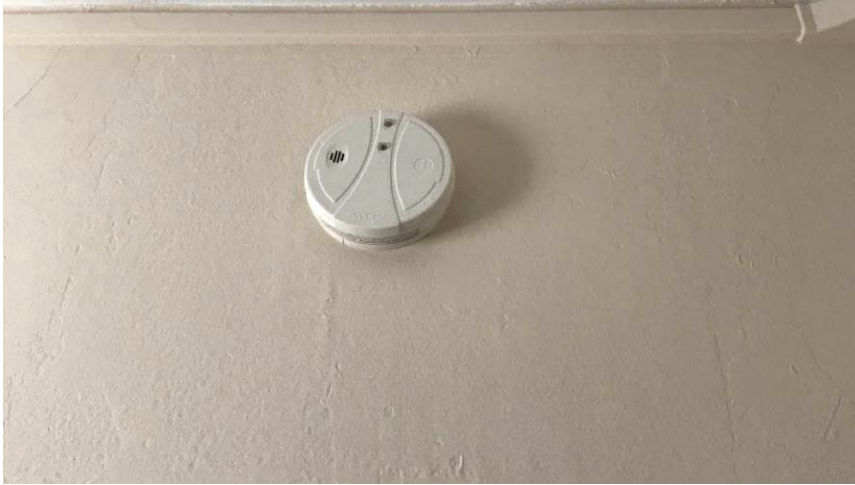
Photo 11: View of radioactive-containing smoke detector observed in Room 206.
