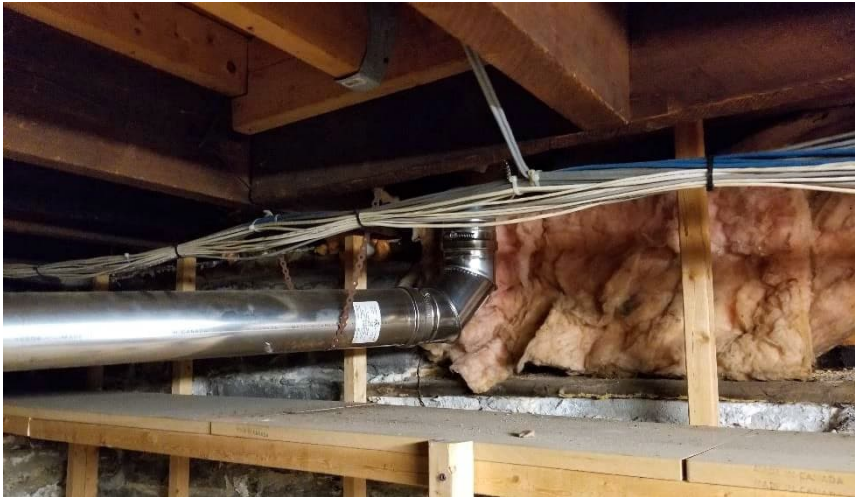
Photo 2: Typical view of finishes in the basement.
