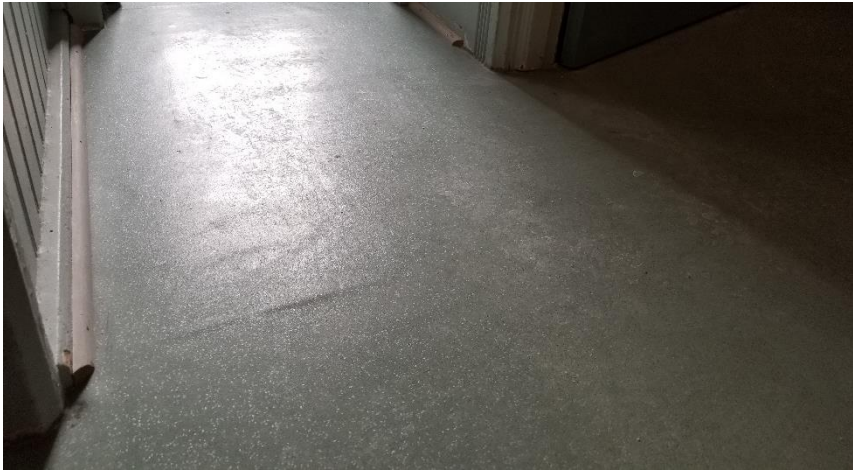
Photo 7: View of non-asbestos vinyl sheet flooring (blue-green) observed in room 203C.
