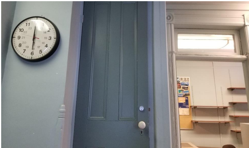
Photo 11: View of lead-containing light blue paint observed on the door of Room 203C
