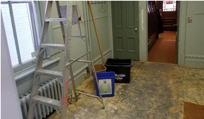
Photo 5: View on non-asbestos carpet mastic (yellow) on the main floor.
