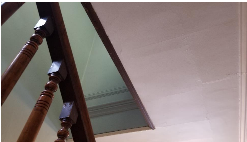
Photo 6: Typical new non-asbestos wall and ceiling plaster on the first floor and stairwell.
