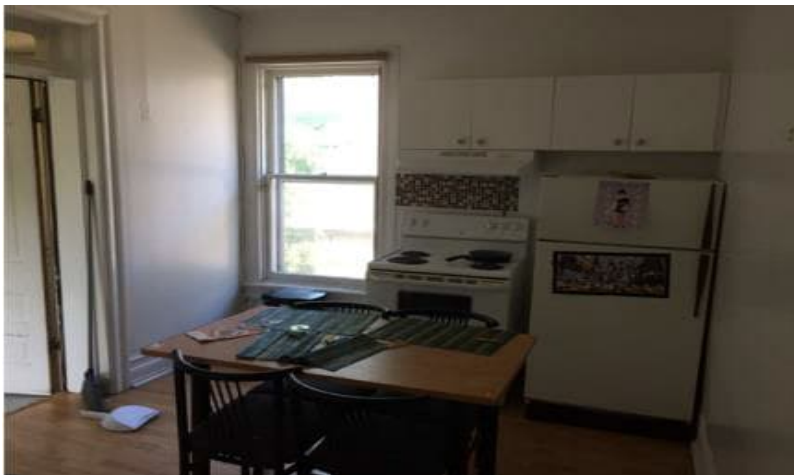
Photo 2: View of typical finishes observed at the building located at 104 Henderson Avenue.
