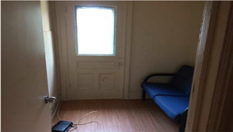
Photo 1: View of typical finishes observed at the building located at 104 Henderson Avenue.
