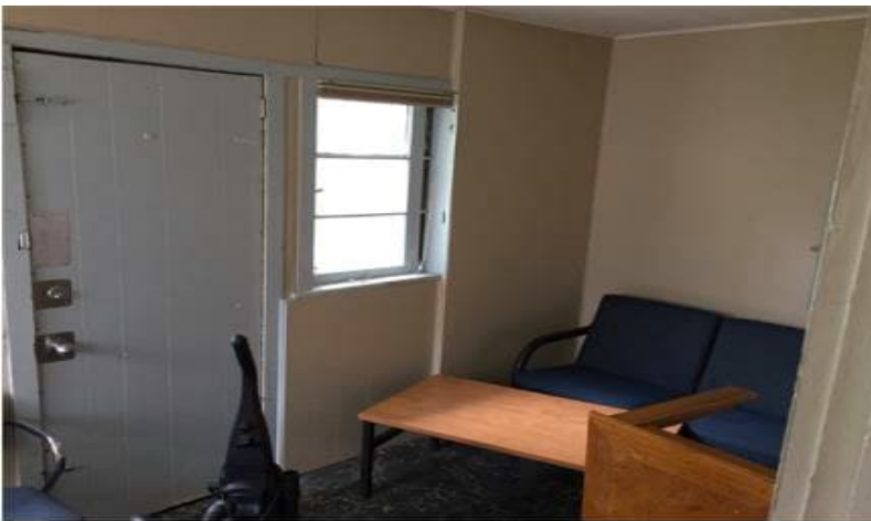
Photo 2: View of typical finishes observed at the building located at 118 Henderson Avenue.
