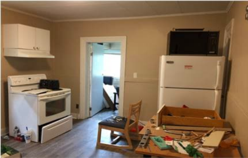
Photo 1: View of typical finishes observed at the building located at 118 Henderson Avenue.
