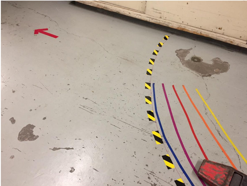
Photo 5: View fair condition grey floor paint with low lead concentration in Room 100C
