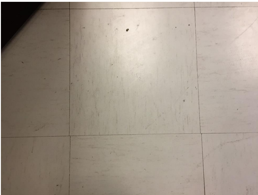
Photo 2: View of asbestos containing VFT – 12"X12" Beige in Room 176
