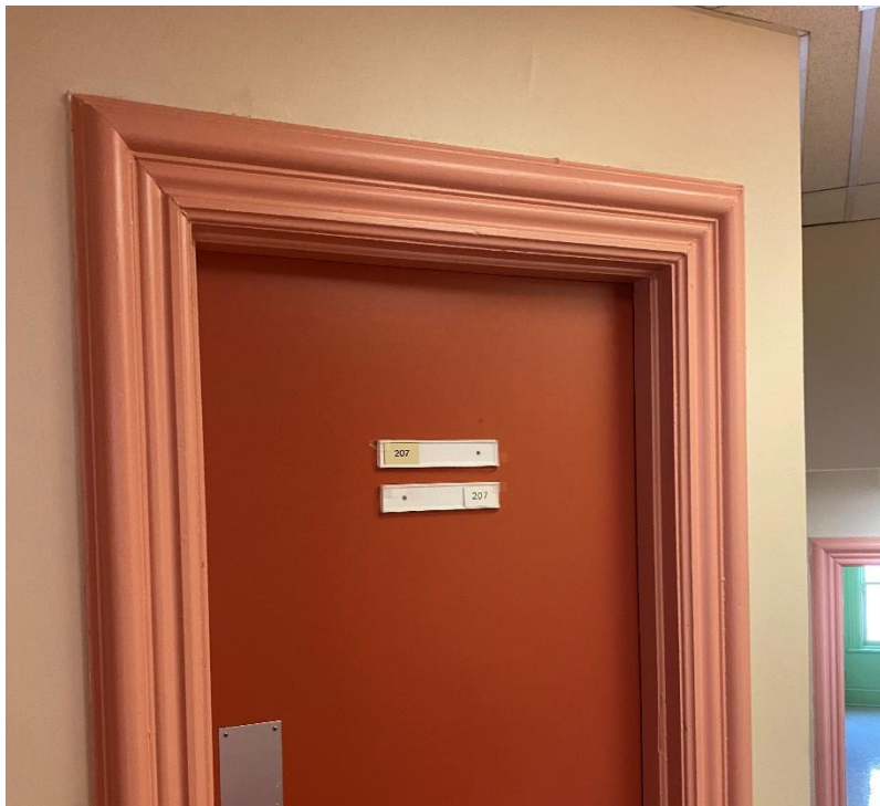
Photo 7: Typical view of paint finishes during the 2023 reassessment near Room 207.
