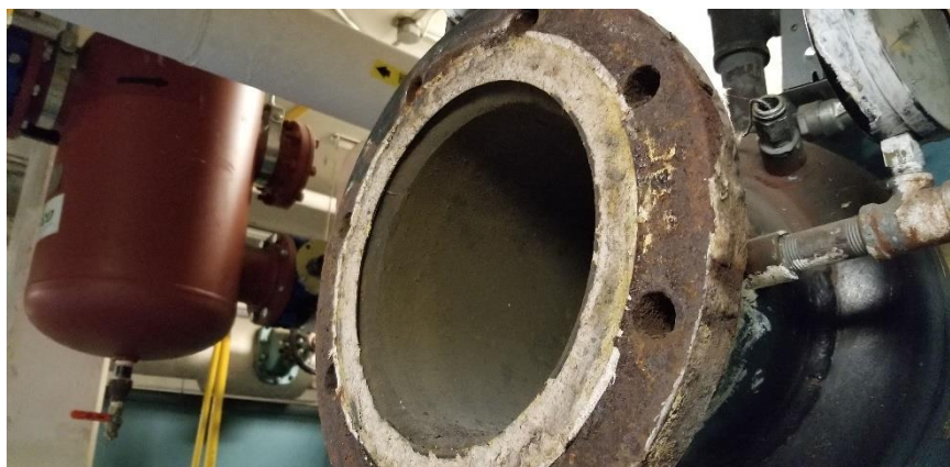
Photo 6: View of asbestos-containing pipe gasket observed on the Unilux Boiler in Mechanical Room A02.
