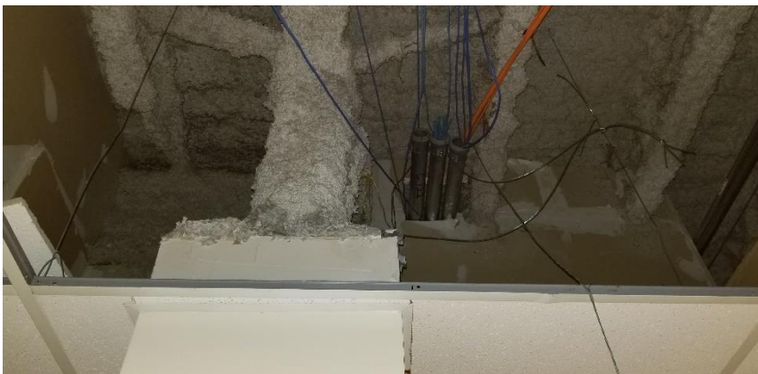
Photo 9: View of non-asbestos containing fireproofing observed above the suspended ceiling tiles in Room C141C.
