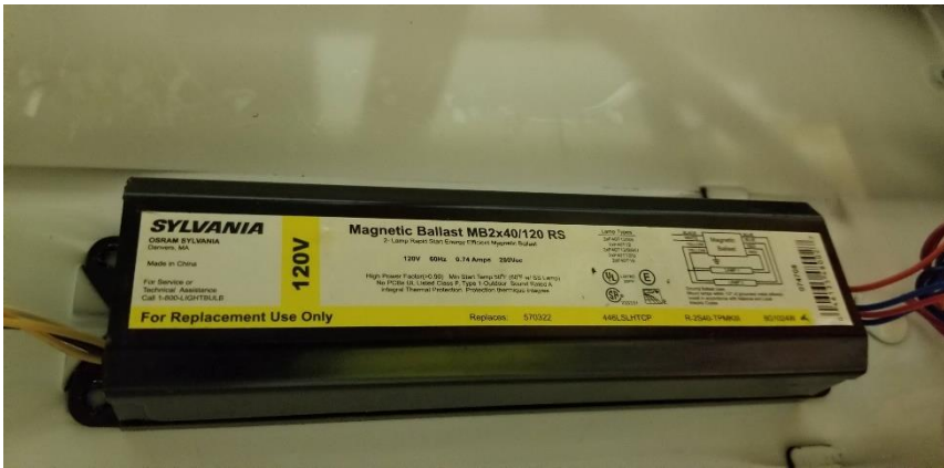
Photo 17: Typical view of non-PCB containing light ballast observed throughout the surveyed building.
