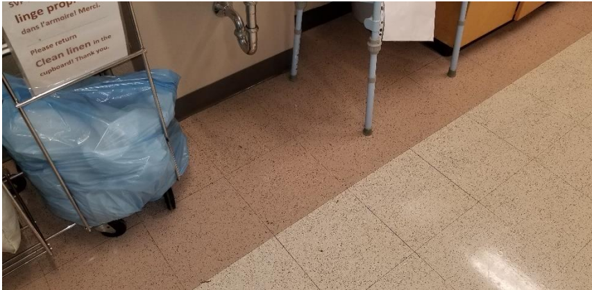
Photo 10: View of non-asbestos containing vinyl floor tiles (12"x12"-Pink with dots) and vinyl floor tiles (12"x12"-Offwhite with dots) observed in Room C115.
