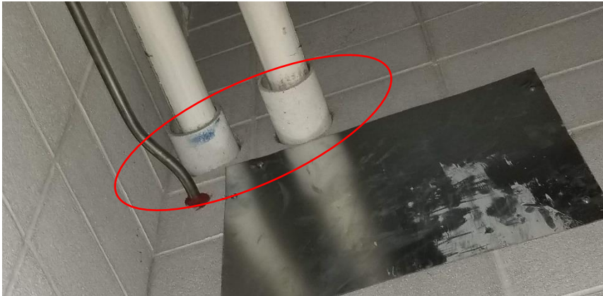
Photo 7: View of asbestos-containing transite pipe (highlighted in red) observed to be in good condition Mechanical Room A138C.
