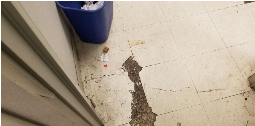
Photo 8: View of asbestos-containing vinyl floor tile (12"x12"-White with beige spots) observed to be in poor condition in Room C144.
