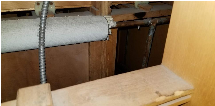
Photo 2: View of asbestos-containing mechanical pipe straight insulation observed to be in poor condition in cabinet 510 in Room A 105.
