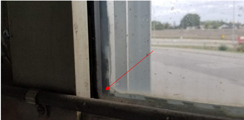
Photo 1: View of asbestos-containing interior window caulking (black) observed to be in good condition in Room 139.
