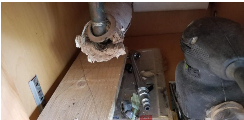
Photo 3: View of asbestos-containing mechanical pipe straight insulation observed to be in poor condition on the 2 nd work bench outside the bike shop office in Room A 105.
