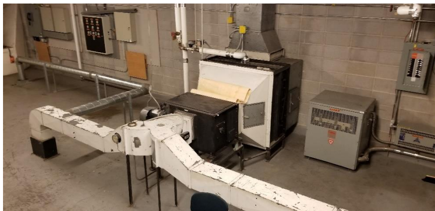
Photo 13: View lead containing white paint observed to be in poor condition in Mechanical Room D201.
