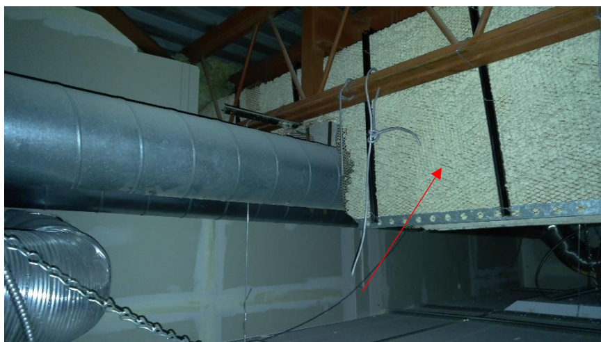
Photo 5: View of asbestos-containing plaster on steel mesh observed in Room B 215N.
