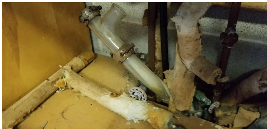
Photo 4: View of asbestos-containing mechanical pipe fittings observed to be in poor condition in Room A104.
