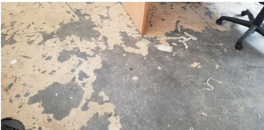
Photo 12: View of low-level lead paint observed to be in poor condition in Room A144.
