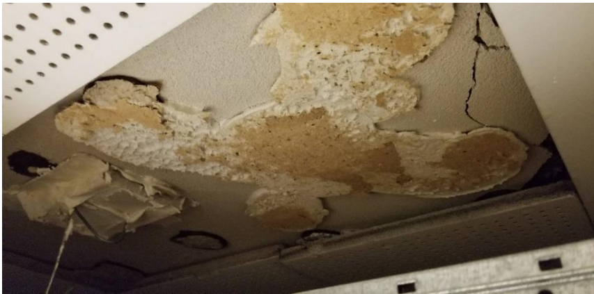
Photo 11: View of non-asbestos containing glued on acoustic tile (12"x12"-Uniform Holes) and adhesive mastic (brown) observed in the Men's Change Room in D108.
