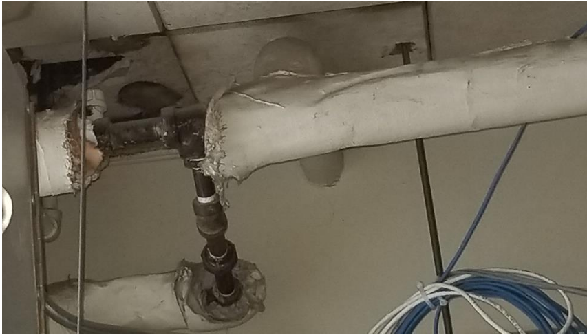
Photo 13: Poor condition asbestos-containing parging cement elbows were observed in Room 010, above suspended ceiling tiles.
