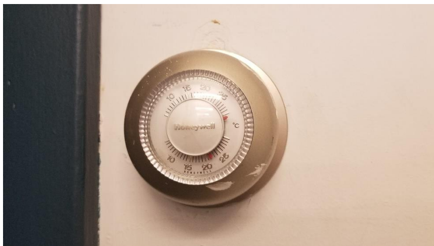
Photo 23: View of Honeywell thermostat containing one ampoule of liquid mercury observed to be in good condition on Room 07.
