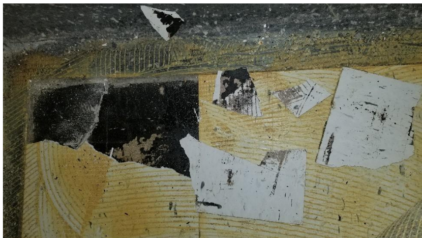
Photo 22: View of asbestos-containing vinyl floor tile mastic (Black) observed to be in good condition on the underside of the carpet in Room 07.
