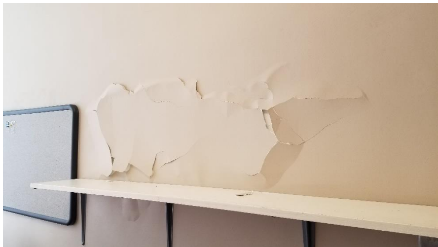
Photo 5: View of the Beige low-level lead wall paint observed in poor condition in Room 111.
