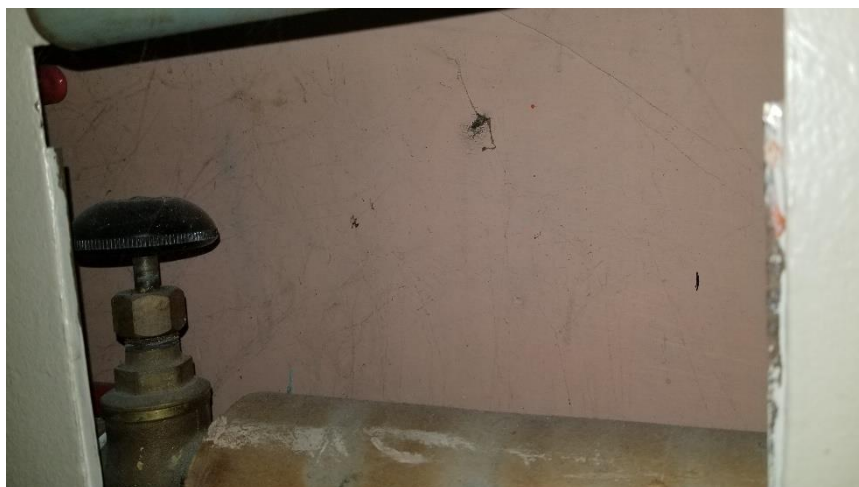
Photo 21: View of the Light Pink paint observed in Room 012, which was determined to contain low levels of lead, and enclosed behind radiator units.
