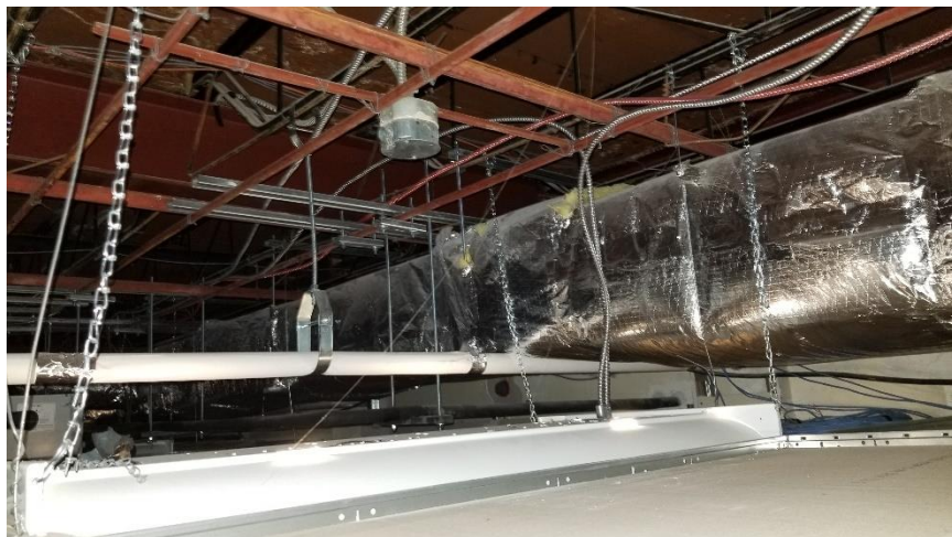
Photo 9: Representative view of the ceiling space throughout Level 1, with visible fiberglass mechanical insulation throughout.
