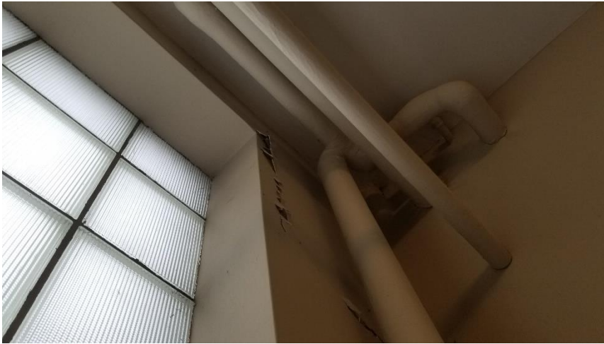
Photo 16: Representative view of the asbestos-containing parging cement elbows observed in good condition in the Women's Washroom Room 013.
