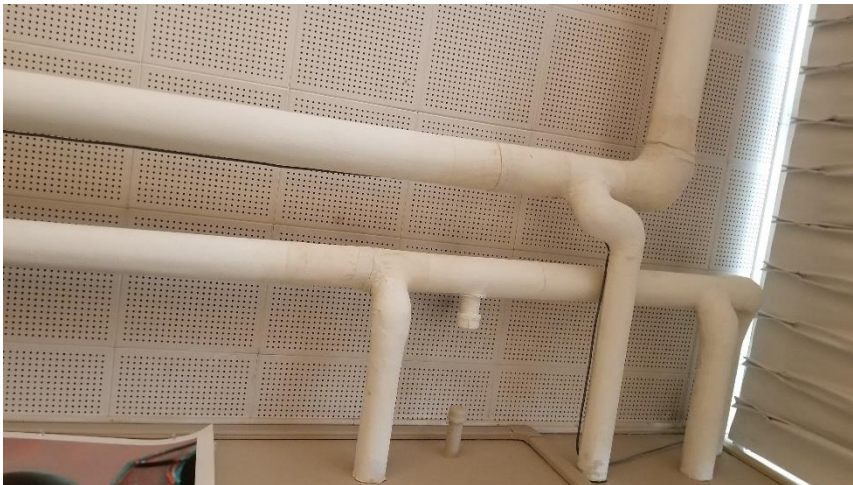
Photo 17: Representative view of the asbestos-containing parging cement elbows observed in good condition in Room 03.
