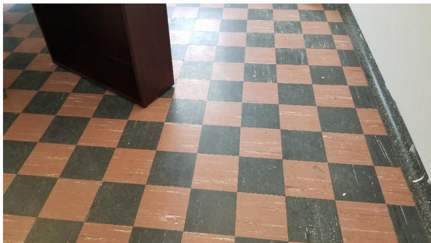
Photo 4: View of the asbestos-containing VFT 9"x9" - Pink & Dark Grey observed in good condition in Room 114B.
