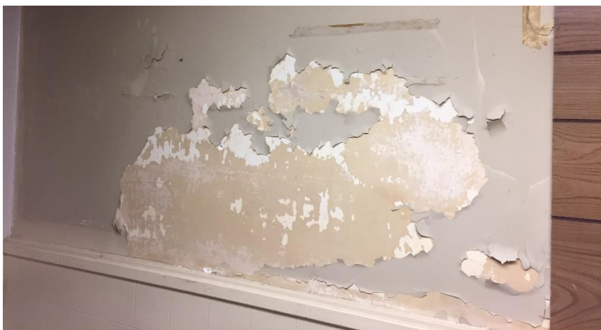
Photo 6: View of the poor condition lead-containing wall paint (Beige) observed in Room B5.
