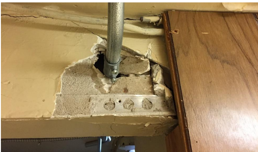
Photo 3: View of the non-asbestos containing wall plaster observed throughout the subject building.
