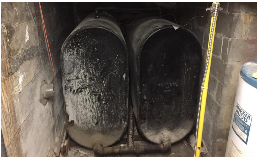
Photo 11: View of the above ground diesel storage tanks identified in Room B8.
