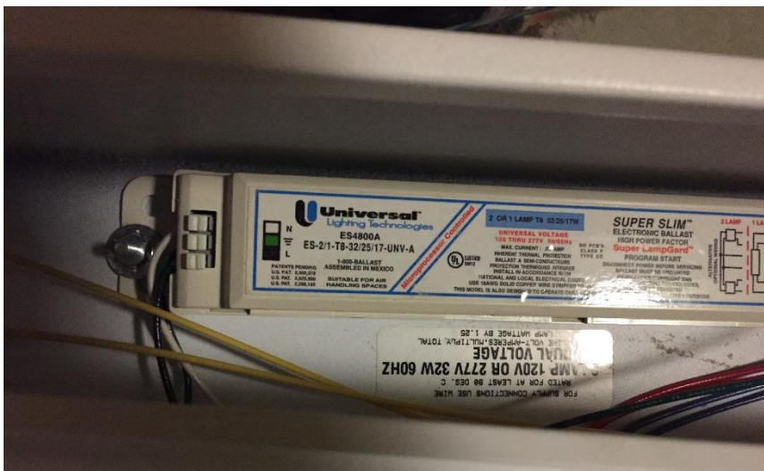
Photo 5: View of the non-PCB light ballasts observed throughout the subject building.
