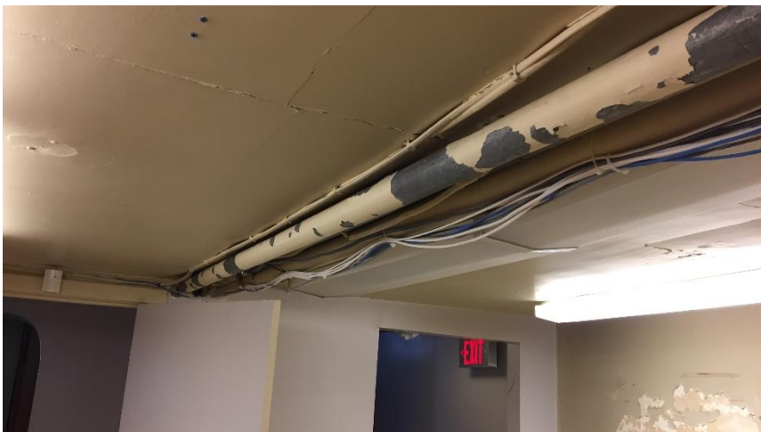
Photo 2: View of the poor condition lead paint (Beige) identified on pipe straights in Room B5.
