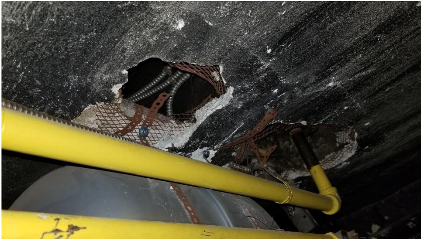
Photo 7: View of the non-asbestos ceiling plaster (Grey) observed in Room B6.
