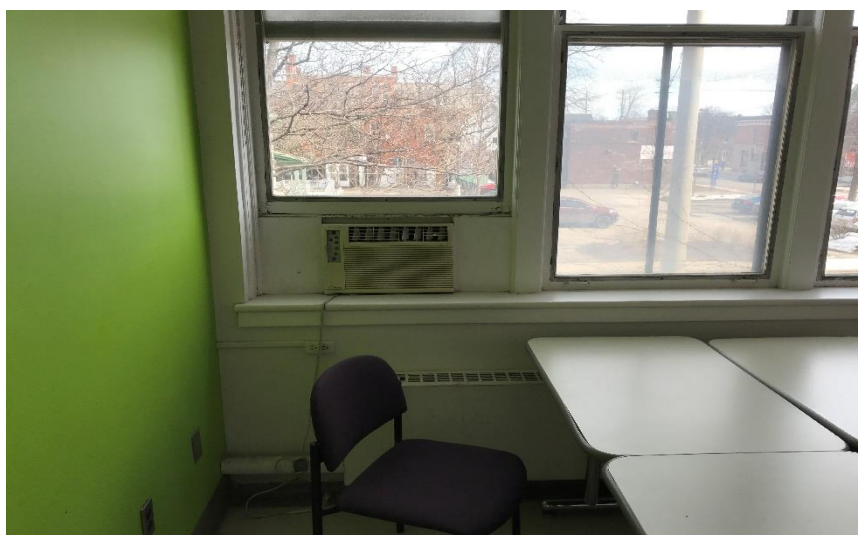
Photo 6: View of air conditioning unit containing ozone-depleted substance in Room 201
