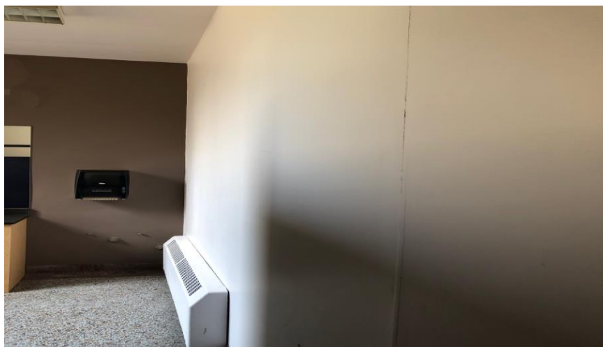
Photo 3: View of asbestos-containing drywall joint compound observed to be in fair condition in Room 202
