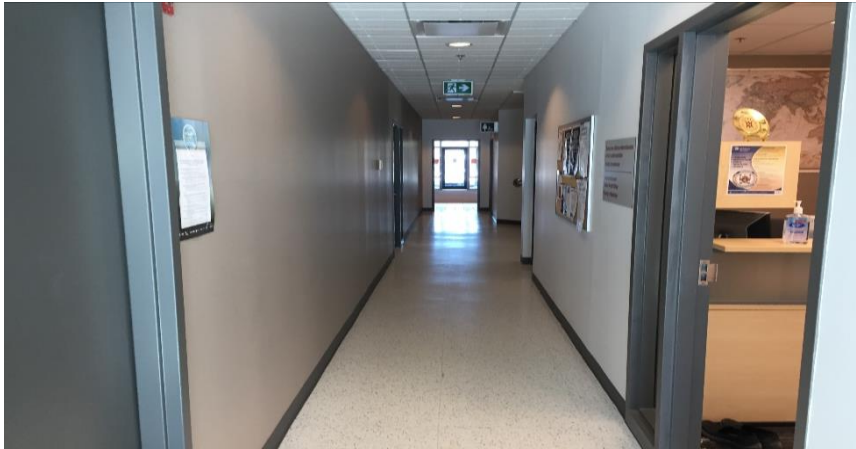
Photo 1: View of typical finishes observed at the building located at 600 Peter Morand Crescent.
