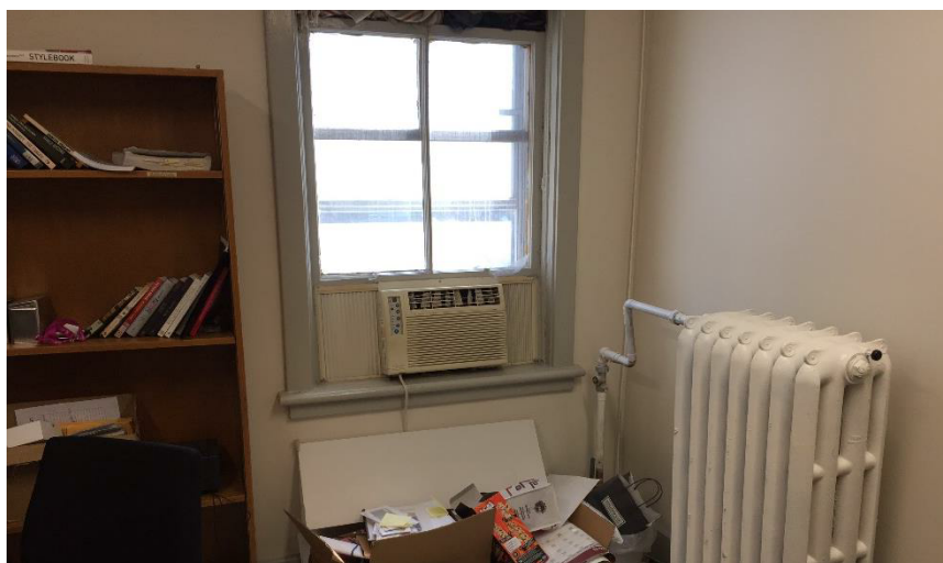
Photo 8: View of the equipment containing ozone depleting substances, observed throughout the subject building.
