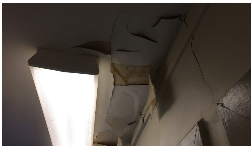
Photo 6: View of the poor condition lead paint (White) and water damaged drywall observed in Room 301
