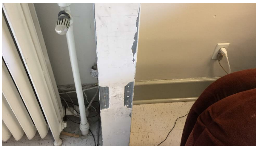
Photo 5: View of the poor condition asbestos-containing drywall joint compound observed in Room 207.
