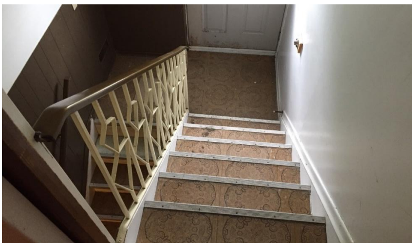
Photo 3: A view of asbestos-containing vinyl floor tiles (Beige with Design) observed in Room 100A.
