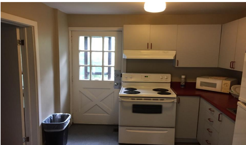
Photo 2: A view of asbestos-containing drywall joint compound and plaster was observed within the subject building.
