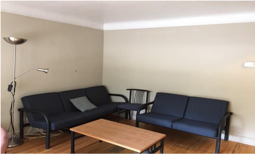
Photo 1: A view of asbestos-containing drywall joint compound and plaster was observed within the subject building.
