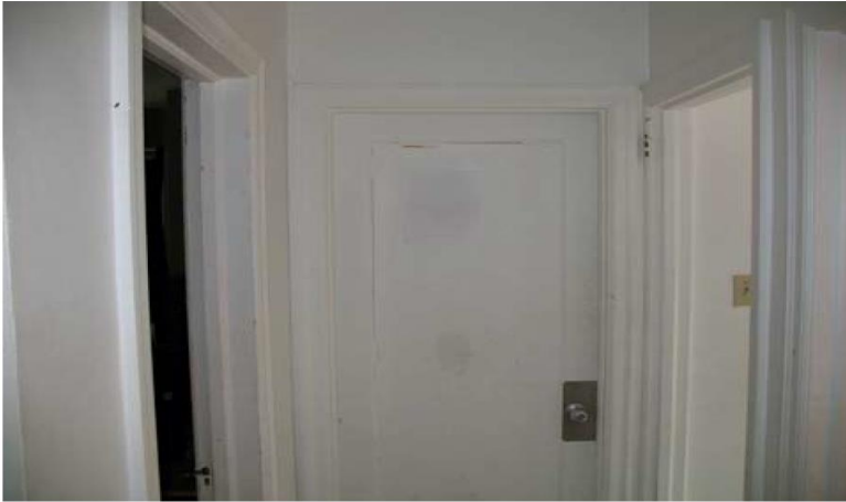
Photo 1: A view of finishes observed at 78 Templeton Street.
