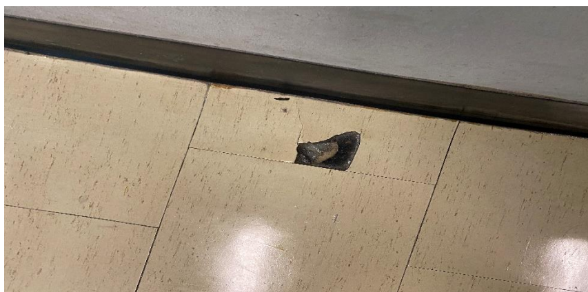
Photo 9: View of fair condition ACM Vinyl Floor Tile (12"x12"-White with Grey Flakes) observed in Location A710.
