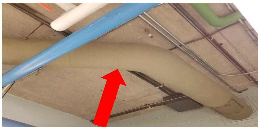
Photo 5: View of asbestos-containing duct insulation observed to be in good condition in Room D320.
