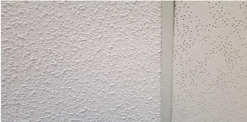
Photo 10: View of non-asbestos ceiling tiles: Pinholes with texture (left) and Pinholes with varying sizes (right) observed in B109C.
