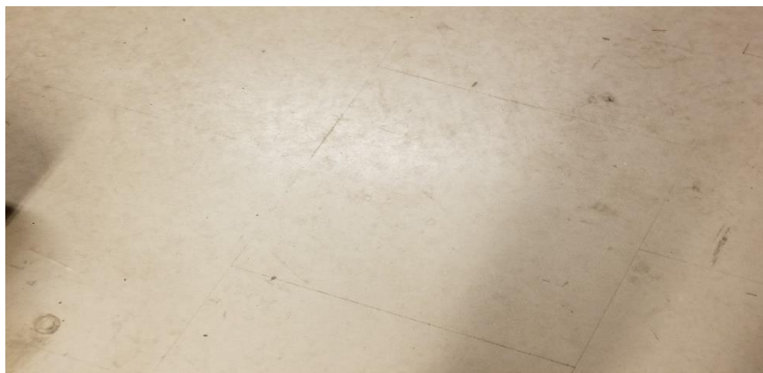
Photo 13: View of non-asbestos containing vinyl floor tiles (12"x12"-Grey ) observed in Room E018B.
