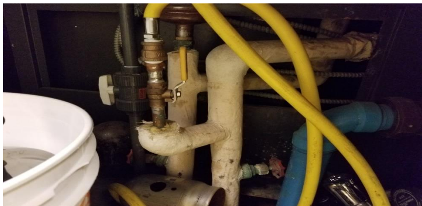
Photo 1: View of asbestos-containing parging cement on fitting observed to be in fair condition underneath the sink in D320.
