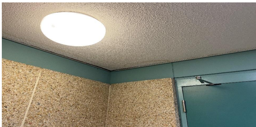
Photo 8: View of poor condition presumed asbestos ceiling texture finish observed in the Hallways outside of A502.
