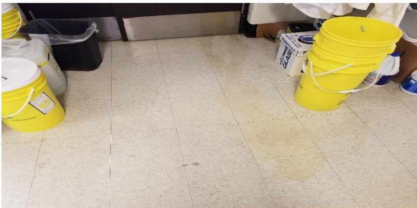
Photo 12: View of non-asbestos containing vinyl floor tiles (12"x12"-White with Grey Flakes) observed in Room D511.
