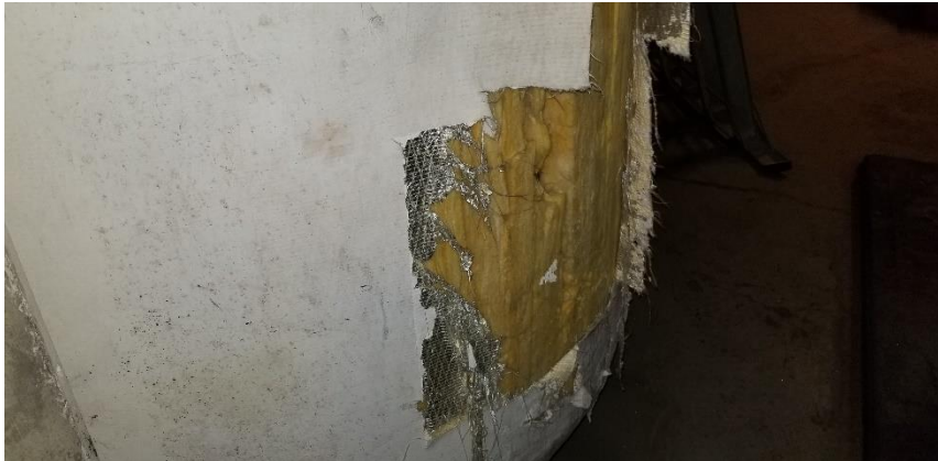
Photo 1: Representative view of the non-asbestos-containing mechanical insulation observed throughout the subject building.
