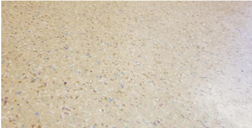
Photo 22: View of the non-asbestos VFT (12"x12" - Pink w/ Multicolour Streaks) observed in Room 223.
