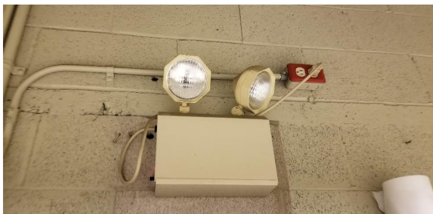
Photo 3: View of the lead battery packs associated with emergency lighting observed in Room 600.
