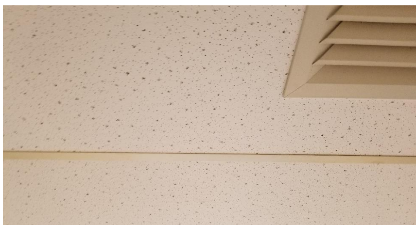
Photo 21: View of the asbestos containing ceiling tiles - 2'x4' Pinholes w/ Triangular Fissures observed in good condition in Room 327.
