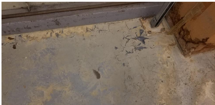
Photo 4: View of the poor condition lead floor paint (Grey) observed throughout Room 600.
