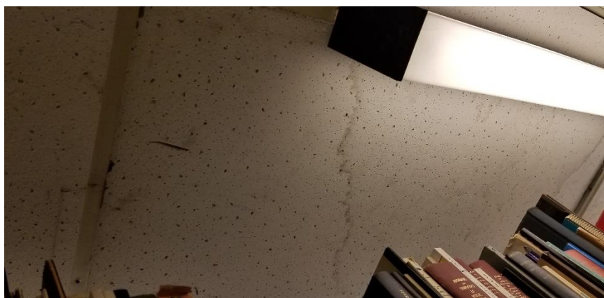
Photo 9: View of the asbestos-containing ceiling tiles - 2'x4' Pinholes w/ Triangular Fissures observed in fair condition in Room 523.
