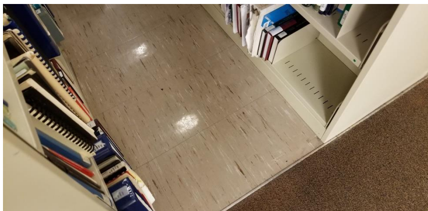
Photo 8: View of the asbestos-containing vinyl floor tiles (12"x12" – Brown w/ Brown Stripes) observed in good condition in Room 523.
