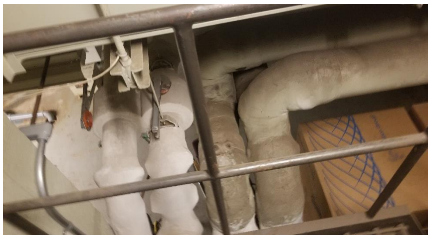
Photo 2: View of the asbestos-containing parging cement elbows observed in good condition throughout Room 600.
