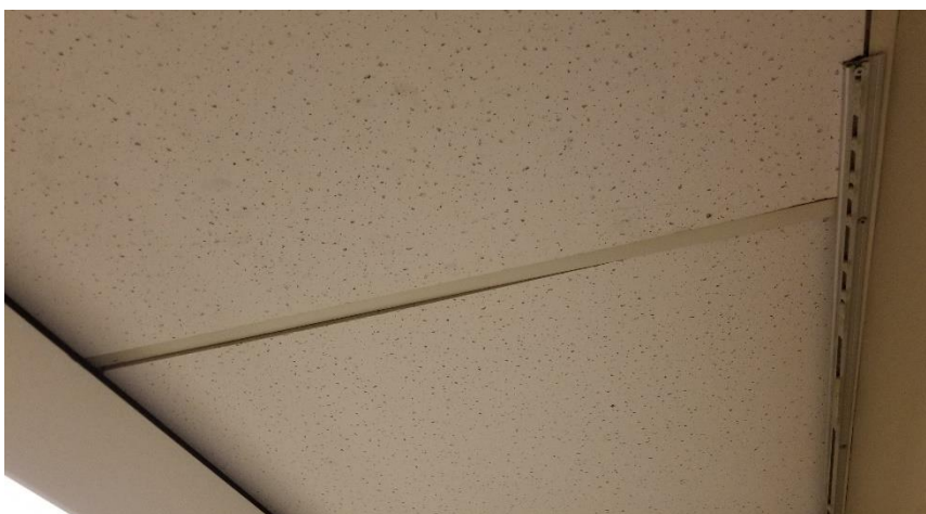
Photo 15: View of the asbestos containing ceiling tiles - 2'x4' Pinholes w/ Triangular Fissures observed in good condition in Room 424.
