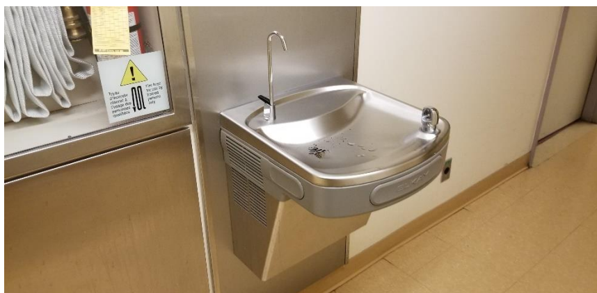
Photo 12: Representative view of the water fountains observed throughout the subject building, containing ODSs.
