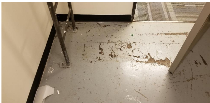
Photo 10: View of the poor condition lead floor paint (Grey) observed throughout Room 525E.
