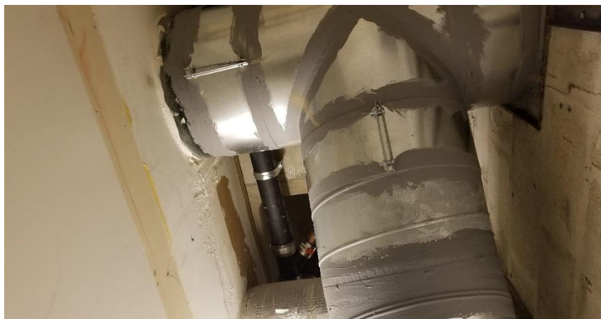
Photo 17: View of the non-asbestos containing caulking (Grey) observed in 371A.
