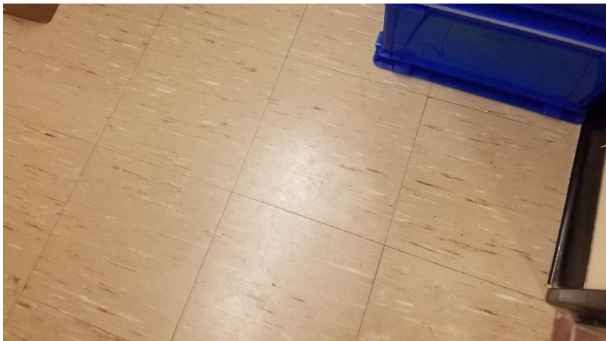
Photo 23: View of the asbestos-containing vinyl floor tiles (12"x12" – Brown w/ Brown Stripes) observed in good condition in Room 224.
