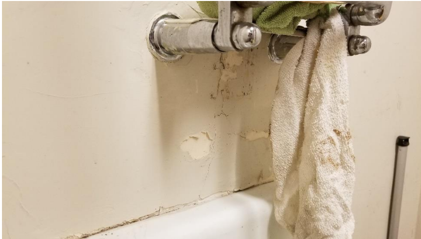
Photo 10: View of the poor condition lead wall paint (Beige) observed in Room 201C.
