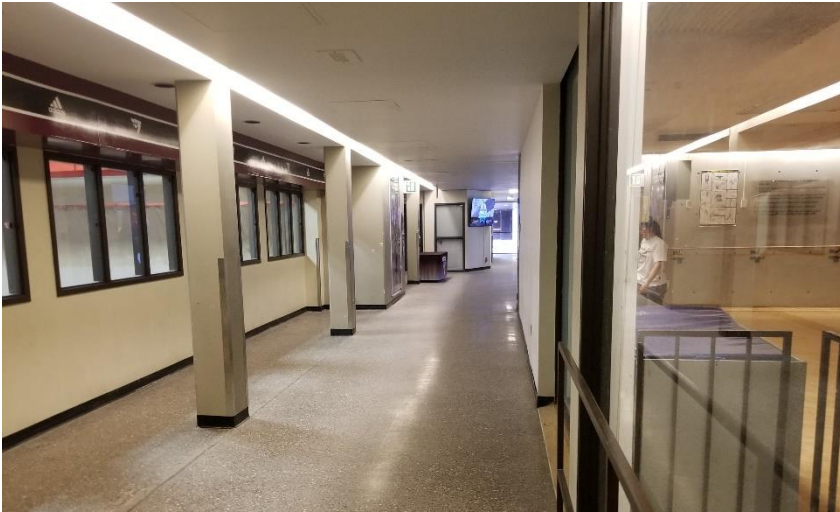
Photo 9: View of typical finishes observed within the subject building.
