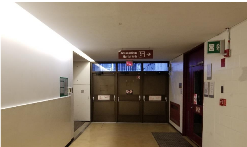
Photo 10: View of typical finishes observed within the subject building.
