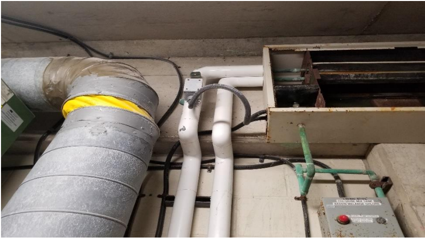
Photo 6: View of flexible duct connector observed in Room 020C suspected to contain asbestos.
