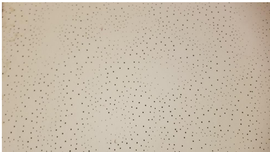
Photo 28: View of the asbestos-containing ceiling tiles (Beige w/ Varying Pinholes) observed and sampled in Room 600G.
