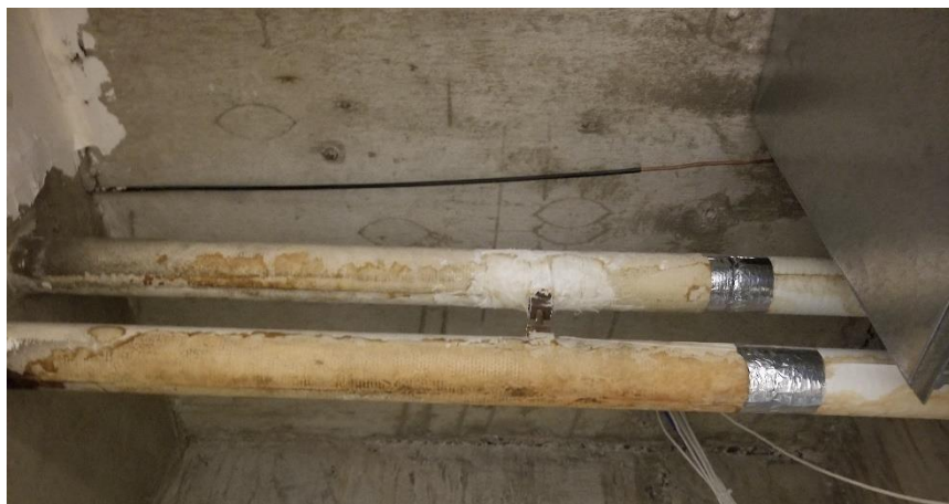
Photo 25: View of the water damaged fiberglass pipe straight insulation observed in Room 510A.
