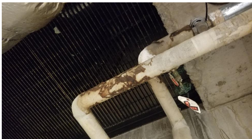
Photo 26: View of the water damaged asbestos-containing parging cement insulation observed in Room 510A.
