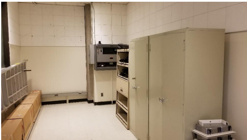
Photo 18: View of the asbestos-containing glue-on acoustic walls tiles observed in good condition in Room 255.
