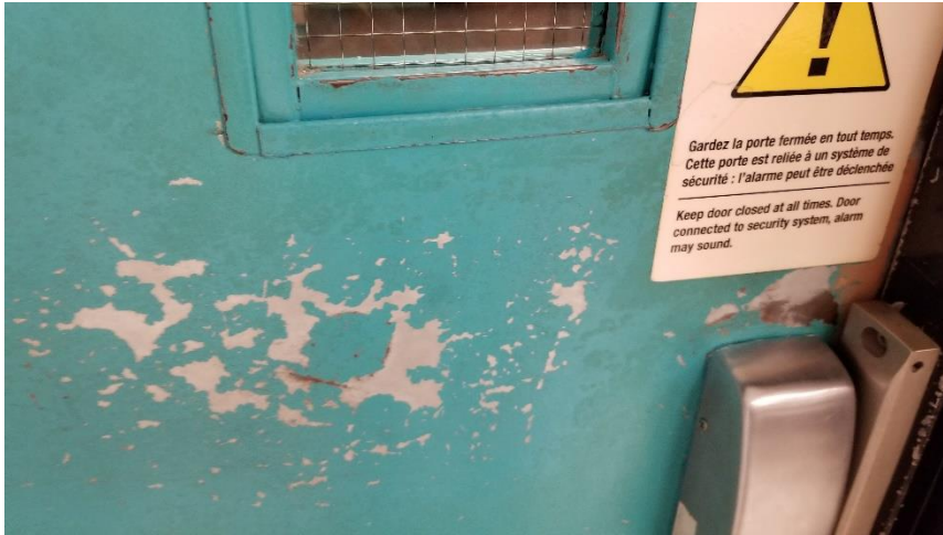
Photo 16: View of the lead containing blue door paint observed in poor condition in Room 217.
