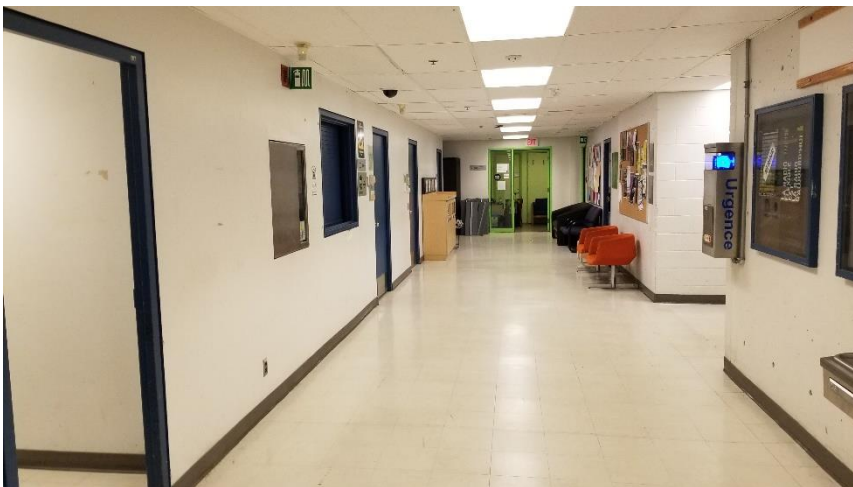
Photo 6: Representative view of Room 001, containing asbestos vinyl floor tiles (12"x12" – White w/ Brown Flakes).
