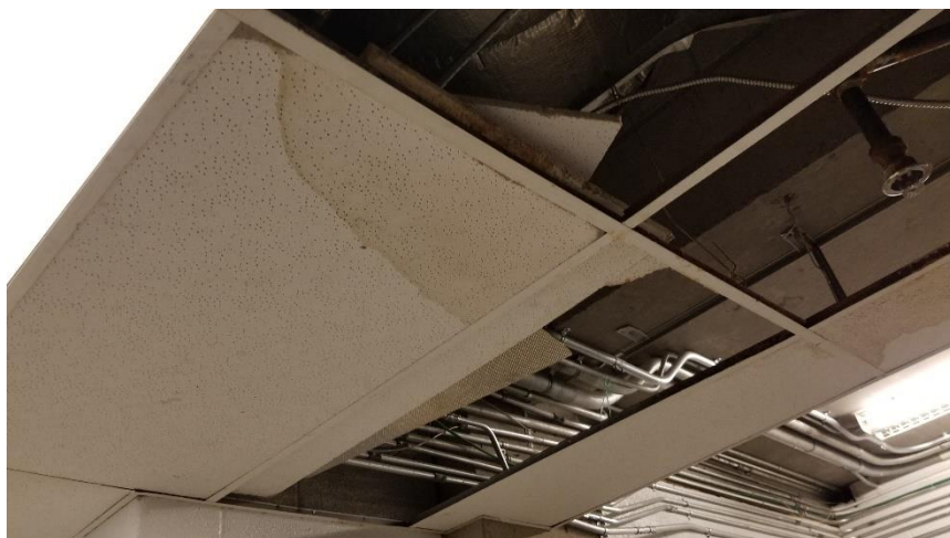
Photo 8: View of the suspended ceiling tiles (2'x4' – Pinholes w/ Large Fissures) observed to be manufactured in 1996 in Room 001A. Water staining was observed on select tiles.
