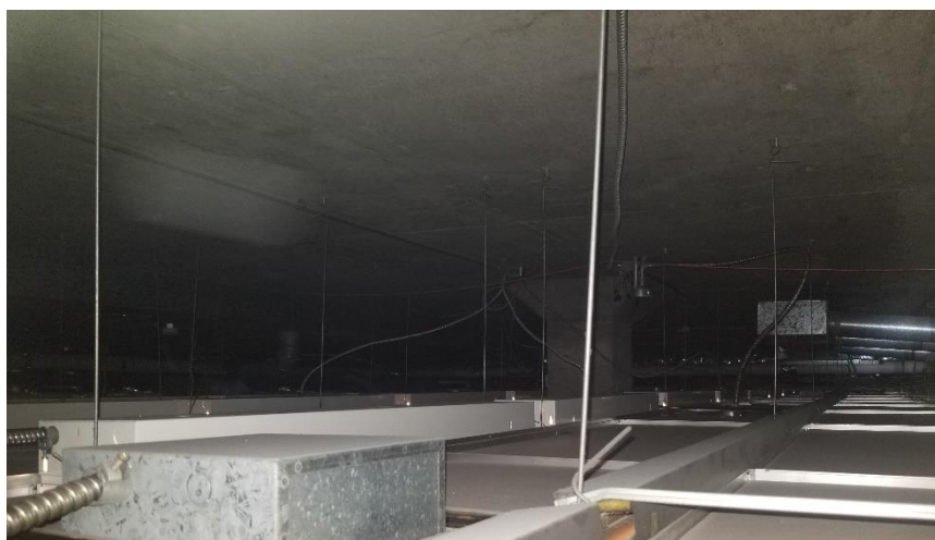
Photo 27: Representative view of the bare concrete ceiling finishes observed above suspended ceiling tiles in Room 600G.
