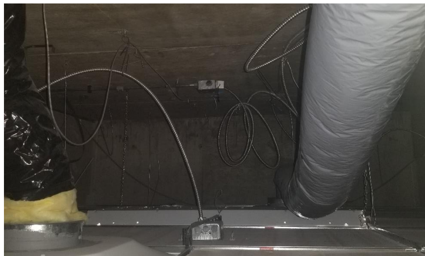
Photo 29: Representative view of the bare concrete ceiling finishes observed above suspended ceiling tiles in Room 602.
