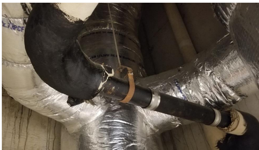
Photo 30: View of the poor condition asbestos-containing pipe straight insulation observed in Room 622A.
