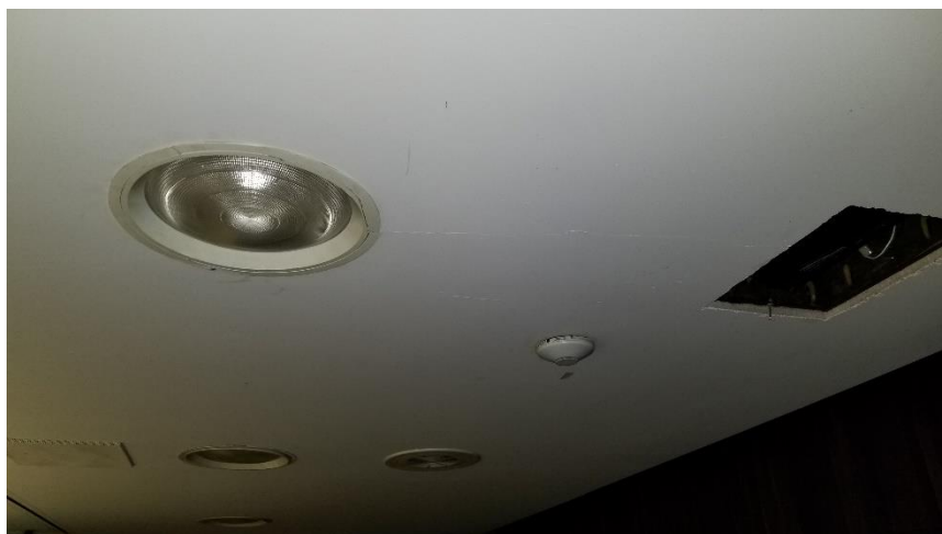
Photo 15: View of the asbestos-containing ceiling plaster observed in Room 218D, with poor condition areas.
