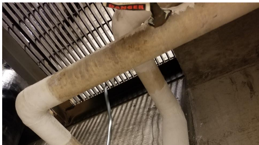
Photo 23: View of the asbestos-containing parging cement elbows observed in good condition in Room 506A.
