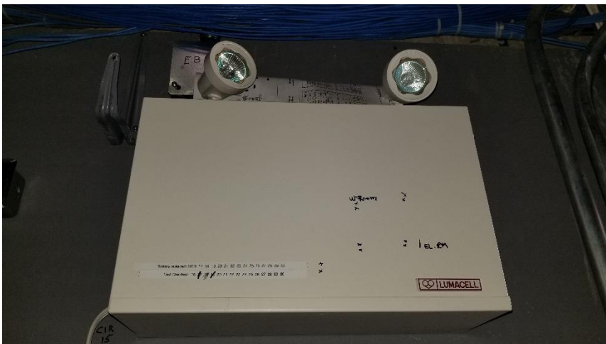
Photo 21: Representative view of the emergency lights containing lead batteries observed in Room 306.
