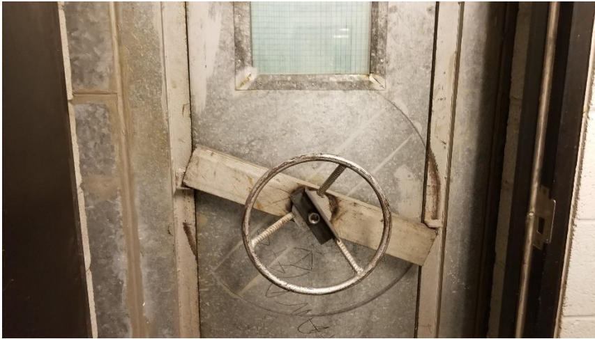
Photo 4: Representative view of the AHU unit doors, with non-asbestos containing thermal insulation in Room 0042.
