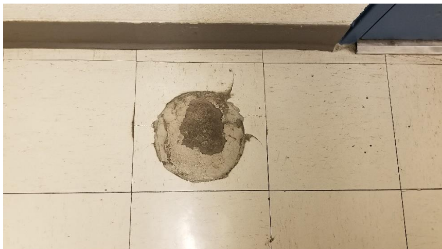
Photo 7: Previously identified vinyl floor tiles (12"x12" – White w/ Brown Flakes) observed in poor condition in Room 001.
