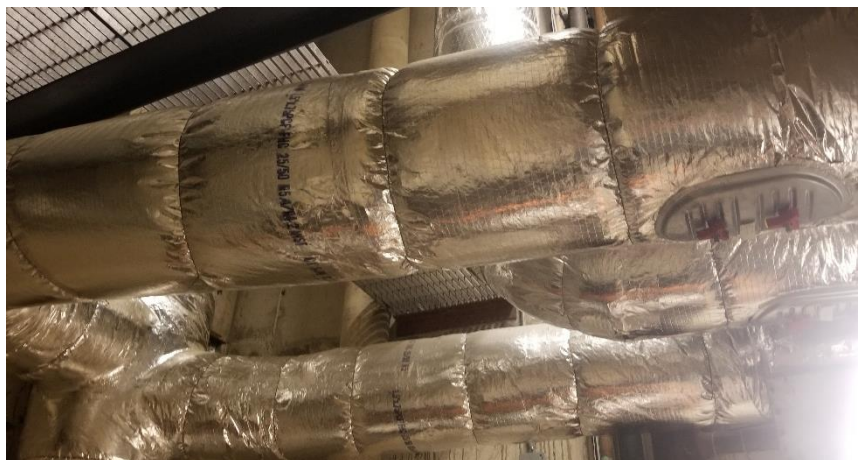
Photo 22: Representative view of the fiberglass insulation observed in Room 431 and 431A.
