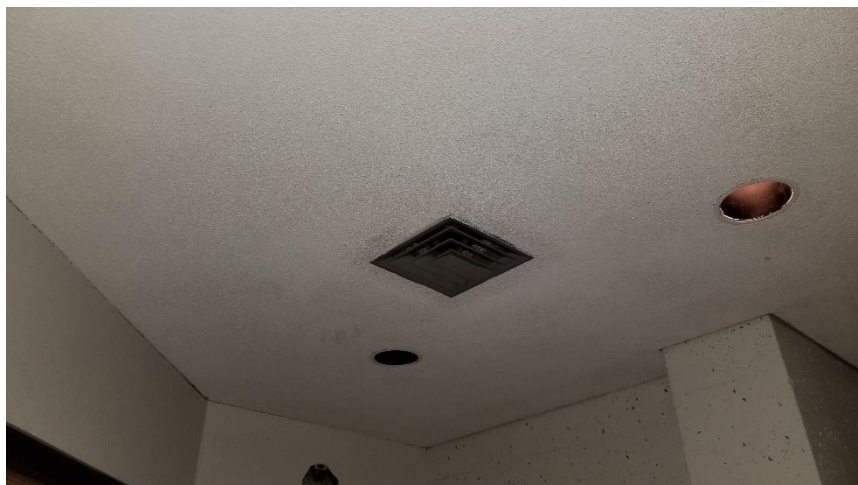
Photo 13: View of the asbestos-containing textured ceiling observed in good condition in Room 218A.
