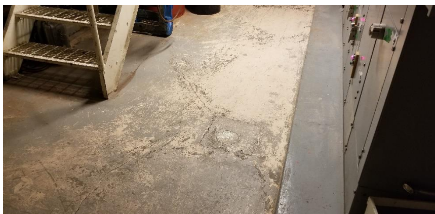
Photo 5: View of the poor condition lead floor paint (Grey) observed in Room 1138.
