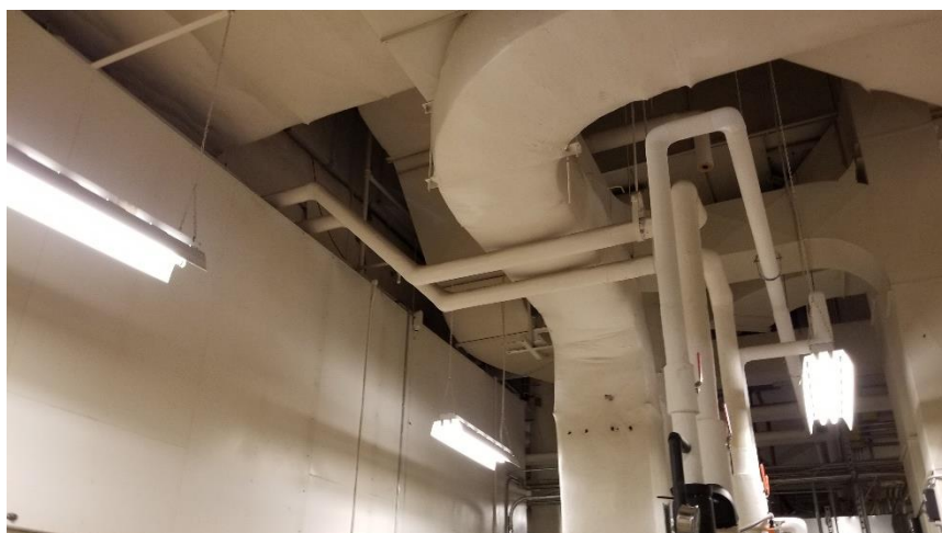
Photo 33: Representative view of the fiberglass mechanical insulation observed in Room 3003B.
