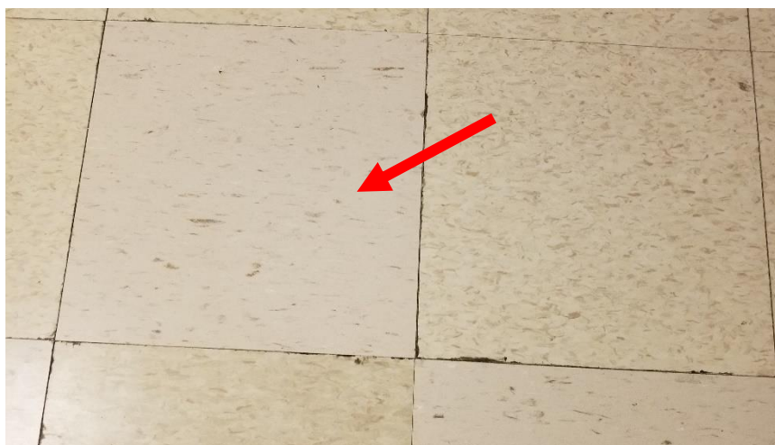
Photo 11: Representative view of the asbestos containing VFT (12"x12" Beige w/ Grey Flakes) observed throughout the subject building.
