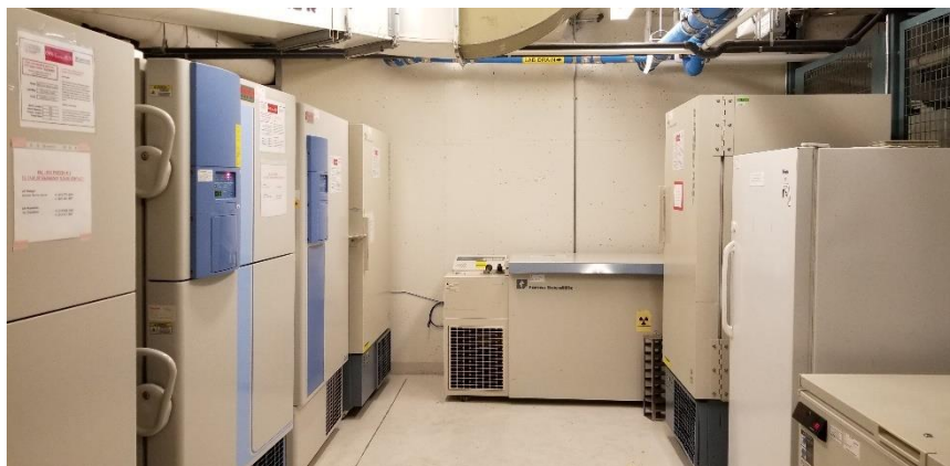
Photo 1: Representative view of refrigeration equipment observed in Room 0509, containing various ozone depleting substances.
