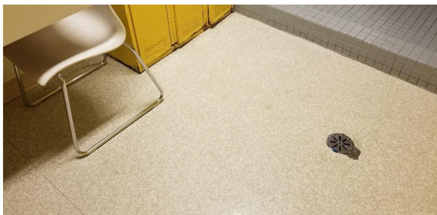
Photo 12: View of the non-asbestos vinyl sheet flooring (Beige Geometric Pattern) observed and sampled in Room 1113.
