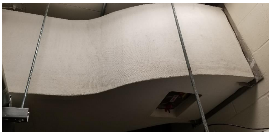
Photo 3: Representative view of the fiberglass insulation observed on HVAC ducts in Room 0515.
