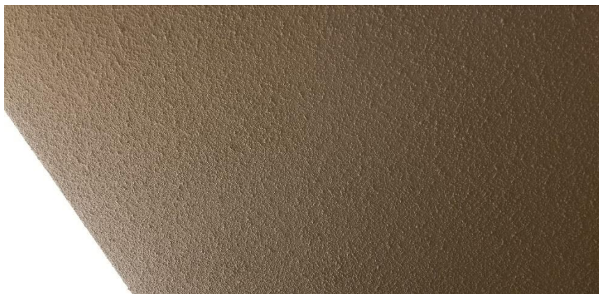
Photo 25: View of the non-asbestos containing ceiling texture coat observed in Room 2213B.
