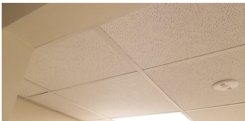
Photo 32: View of the non-asbestos containing ceiling tiles (2'x4' Mixed Pinholes) observed in 3105T and manufactured in 2016 and 2017.
