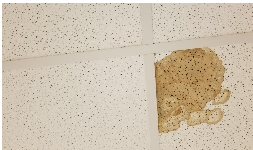
Photo 35: Representative view of water damaged ceiling tiles observed throughout the subject building.
