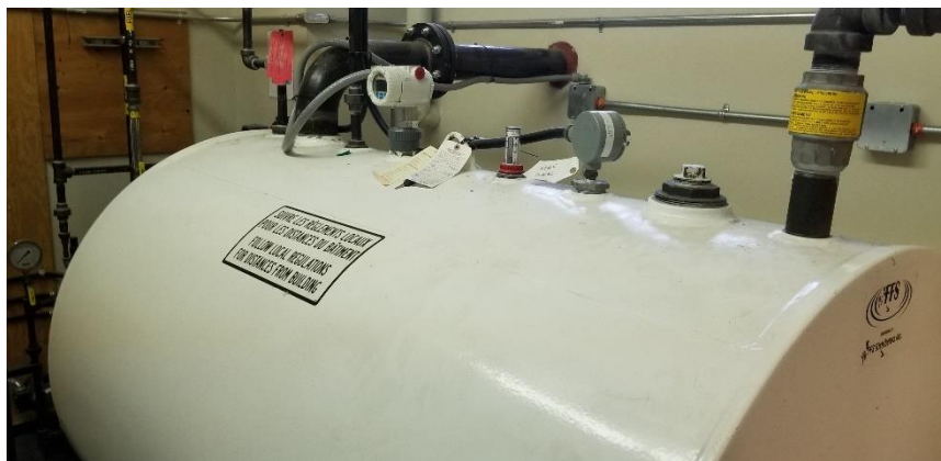
Photo 7: View of the above ground diesel storage tank observed in Room 1129C.
