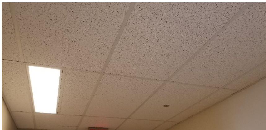
Photo 37: View of the non-asbestos ceiling tiles (2'x4' – Pinholes & Small Fissures) observed in Room 4200A.
