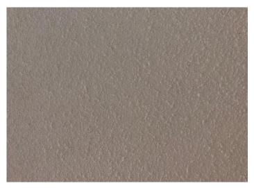
Photo 8: View of asbestoscontaining texture coat observed in Room 1608.
