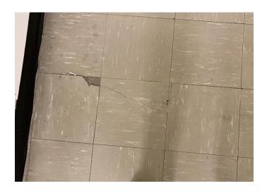
Photo 10: View of asbestoscontaining vinyl floor tiles (12"x12"grey with white streaks) observed in fair condition in Room 130F.
