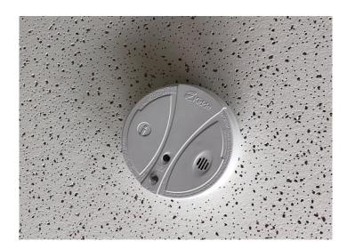
Photo 16: Typical view of smoke detectors containing radioactive materials.
