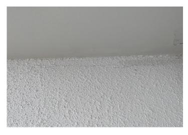
Photo 12: View of asbestoscontaining texture coat observed in fair condition in Room 1607.
