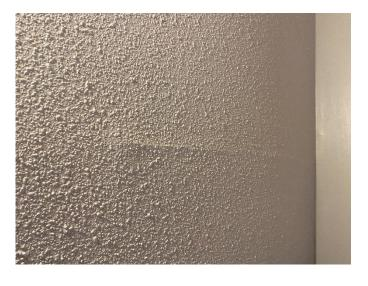
Photo 9: View of asbestoscontaining texture coat observed in fair condition in Room 130F.
