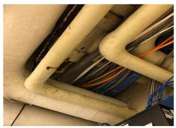
Photo 14: View of asbestoscontaining pipe fitting insulation observed in Room 025.
