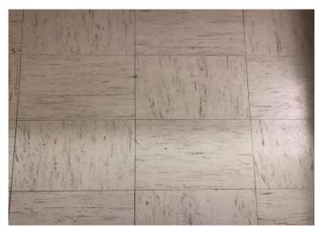
Photo 5: View of asbestoscontaining vinyl floor tiles (12"x12"- white with grey streaks) observed in Room 1618A (kitchen).
