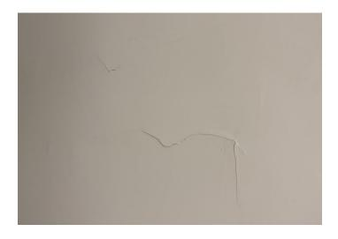
Photo 13: View of asbestoscontaining drywall joint compound observed in fair condition in Room 1607.
