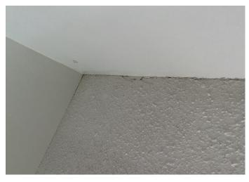
Photo 11: View of asbestoscontaining texture coat observed in fair condition in Room 312.
