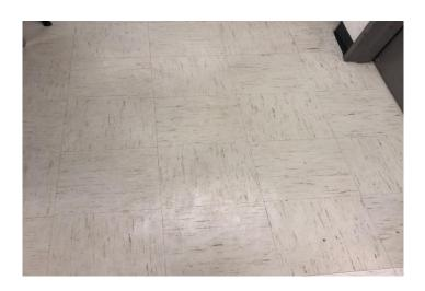
Photo 7: View of asbestoscontaining vinyl floor tiles (12"x12"- white with black streaks) observed in Room 017.
