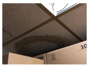
Photo 17: View of water damaged ceiling tiles observed in Room 100G.
