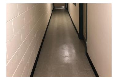
Photo 6: View of asbestoscontaining vinyl floor tiles (12"x12"- grey with white streaks) observed in the basement corridor.
