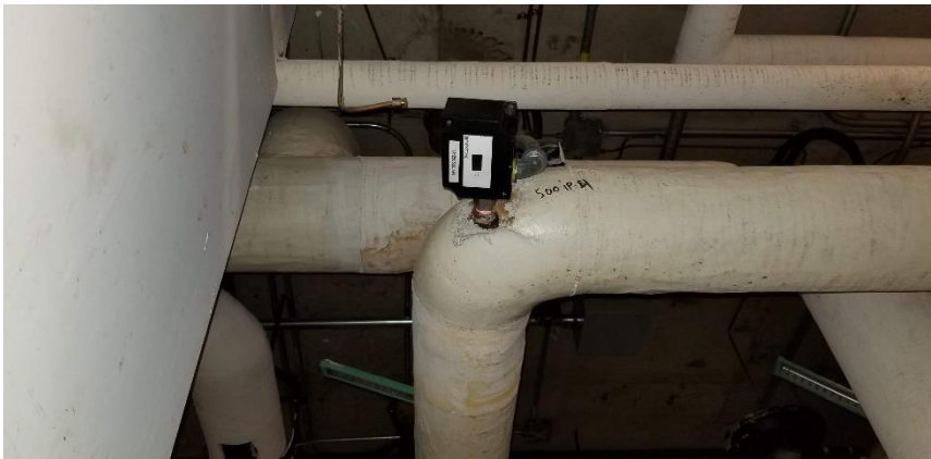
Photo 6: View of asbestos-containing parging cement on pipe fitting observed to be in poor condition in Room 0033H.
