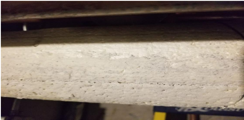
Photo 8: View of asbestos-containing parging on foam pipe insulation observed to be in good condition in Room 0027.
