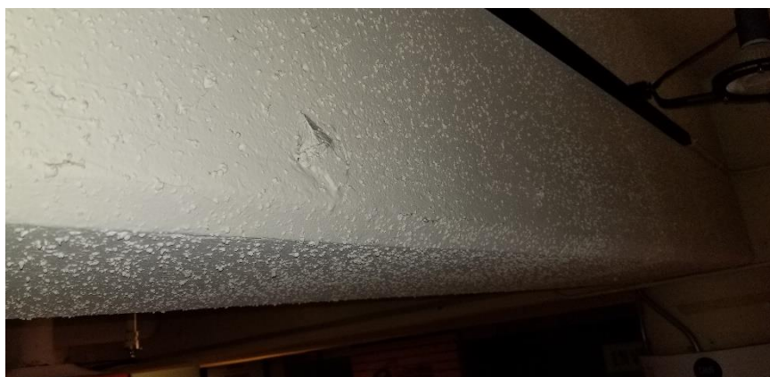
Photo 14: View of non-asbestos containing ceiling texture coat observed on the concrete ceiling deck in the common area 031.
