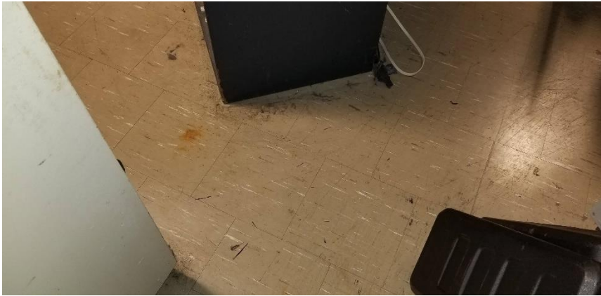
Photo 1: View of asbestos-containing vinyl floor tiles (12"x12"-Beige with White and Brown Flakes) observed to be in good condition in Room 100G.
