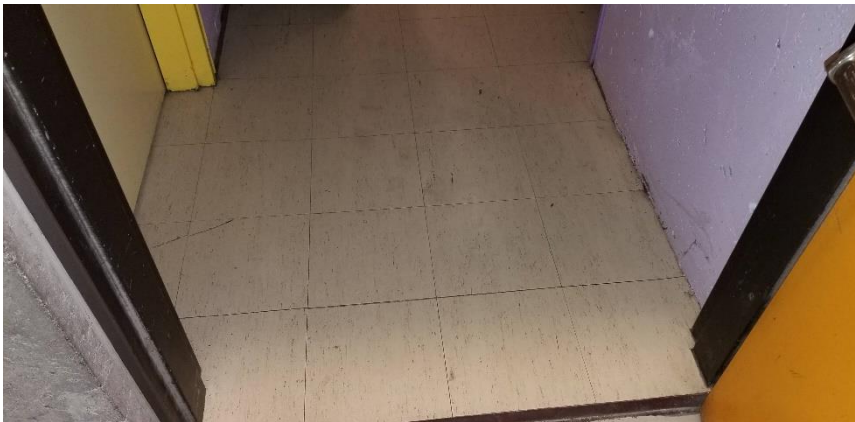
Photo 9: View of previously identified asbestos-containing vinyl floor tiles (12"x12" - Beige with Brown Spots) observed to be in good condition in the hallway of 002 and in adjacent rooms.
