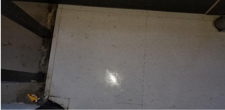
Photo 10: View of asbestos-containing vinyl floor tiles (12"x12"-Beige with Gray Flakes) observed to be in good condition at the A03 stairwell landing.
