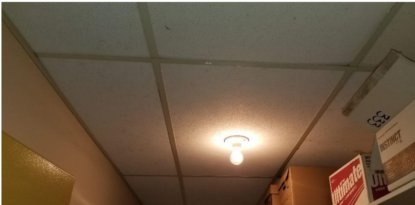
Photo 12: View of asbestos-containing suspended ceiling tiles (2'x4'-White with dots) observed to be in Room 333B.
