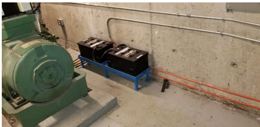
Photo 20: View of lead containing acid batteries observed to be in good condition in Room 0033H.
