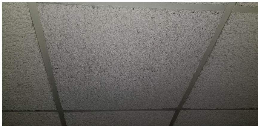
Photo 16: View of non-asbestos containing suspended ceiling tiles (2'x2'-Deep Texture) observed in 014 Hallway.
