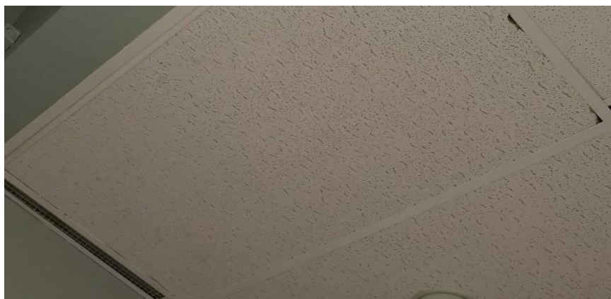
Photo 17: View of non-asbestos containing suspended ceiling tiles (2'x4'-Pinholes with Large Fissures) observed in Room 211.
