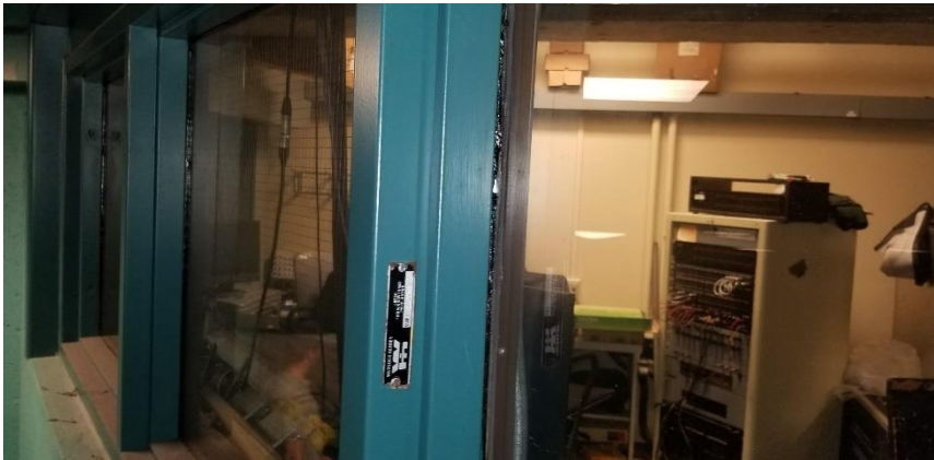
Photo 2: View of asbestos-containing window caulking (Black) observed to be in good condition outside of Room 100G.
