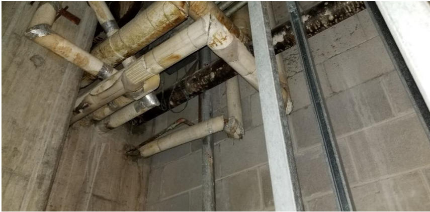
Photo 7: View of asbestos-containing mechanical pipe straight insulation (AirCell) observed to be in poor condition in Room 0033B.
