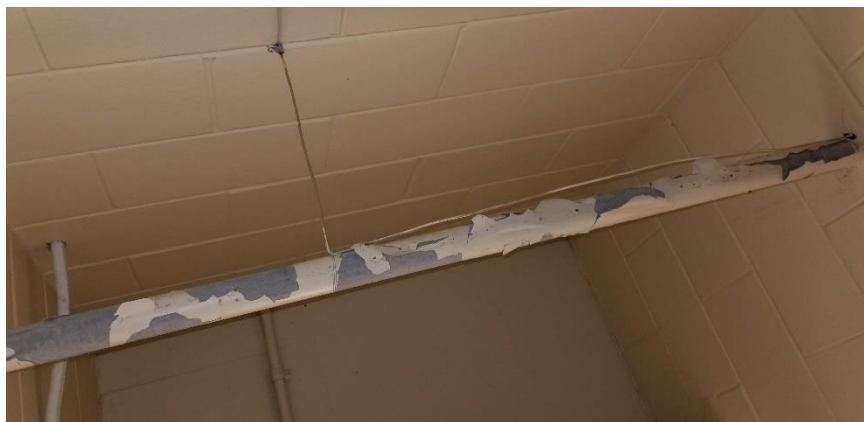
Photo 19: View of lead paint finish (Off-White) observed to be in poor condition on a mechanical pipe in Room 017.
