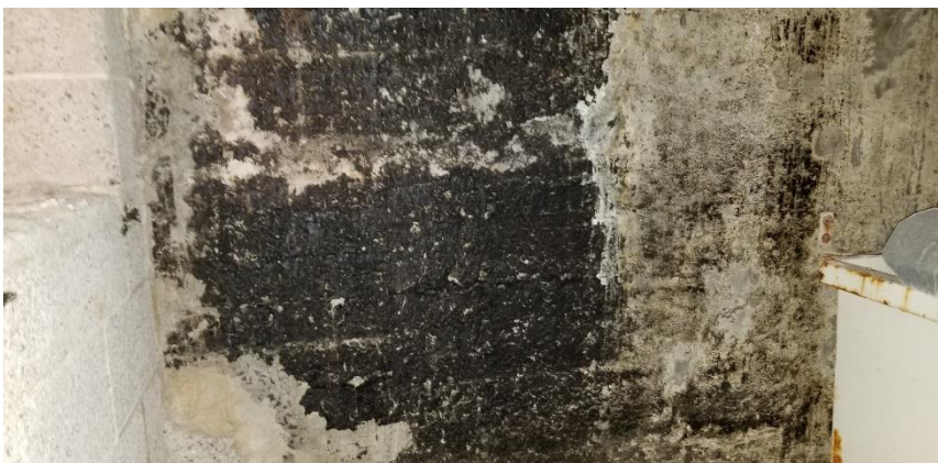
Photo 9: View of non-asbestos containing wall mastic (Black) observed in Room 0140.
