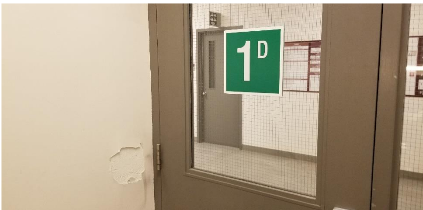
Photo 5: View of asbestos-containing wall plaster observed to be in poor condition in Room 1070.
