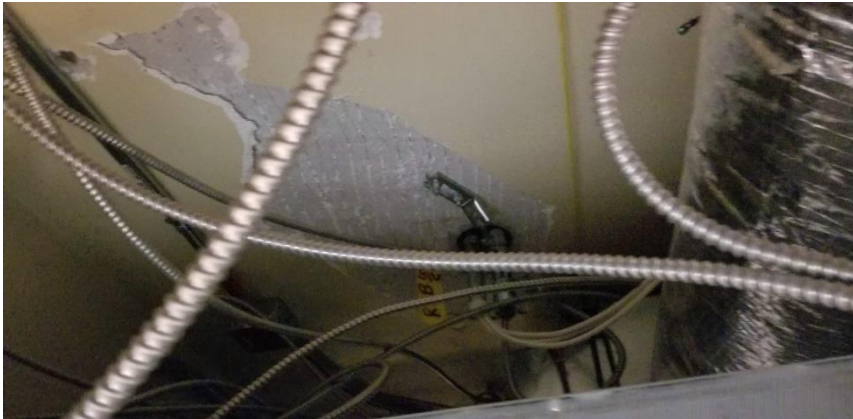
Photo 4: View of asbestos-containing ceiling plaster observed to be in poor condition above the suspended ceiling tiles in Room 1026.
