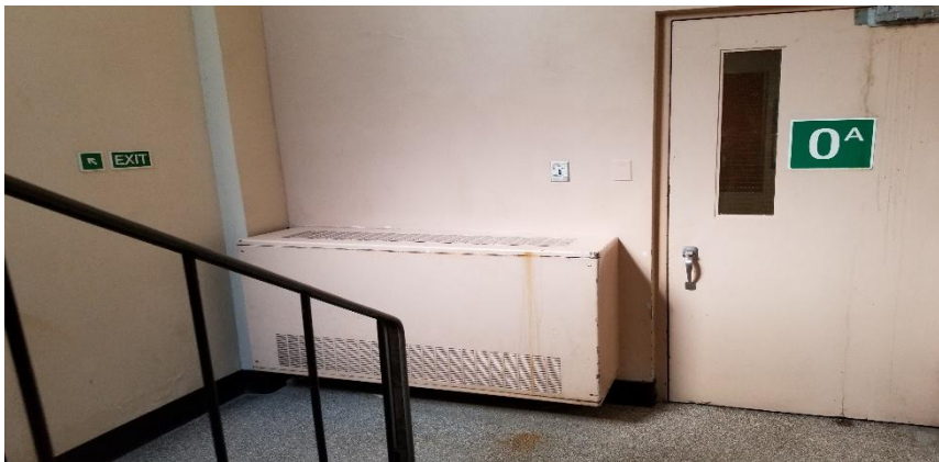
Photo 13: Typical view of low-level lead containing pink paint finish observed to be in good condition on radiators and walls throughout the subject building.
