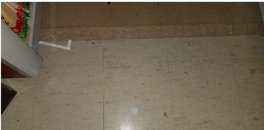
Photo 2: View of asbestos-containing vinyl floor tiles (12"x12"-Cream and Brown Coloured) observed to be in good condition in Room W0041.
