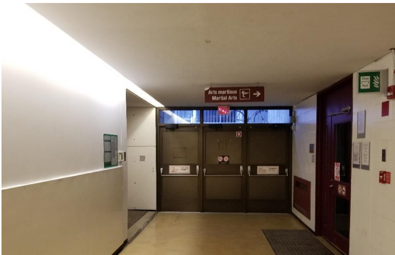
Photo 10: View of typical finishes observed within the subject building.
