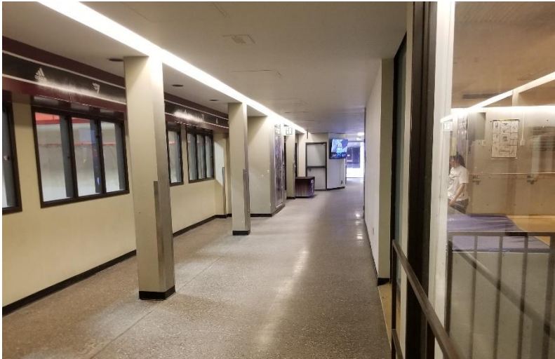
Photo 9: View of typical finishes observed within the subject building.
