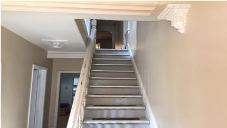
Photo 1: View of typical finishes observed at the building located at 112 Henderson Avenue.
