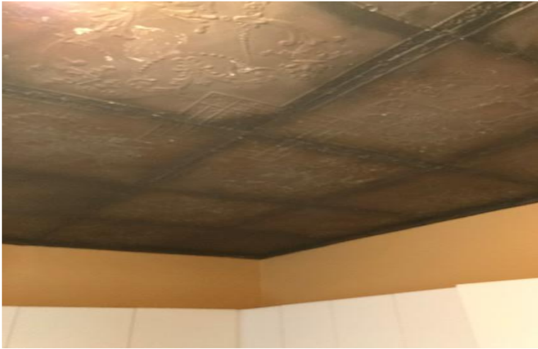
Photo 1: View of finishes observed in the kitchen at 134 Henderson Avenue.
